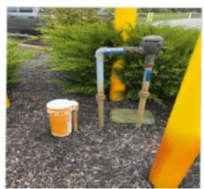
4 A Minor deficiency was identified regarding: Cross connection(s) in the treatment process
