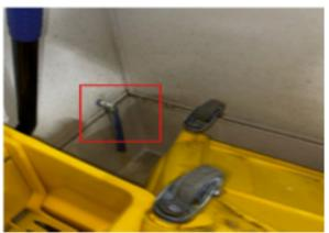
4 A Minor deficiency was identified regarding: Cross connection control devices are not properly installed, tested, or inspection
