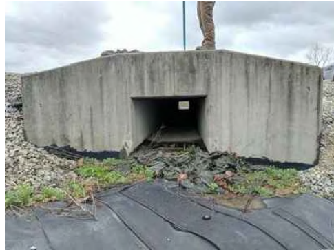
PHOTO 1 EXISTING CONCRETE CULVERT (UPSTREAM END)
