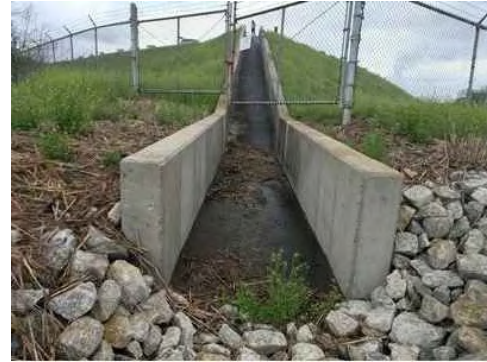
PHOTO 2 EXISTING CONCRETE CHUTE
