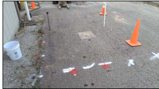
Photo 2: S – Injection point layout (red locations)
