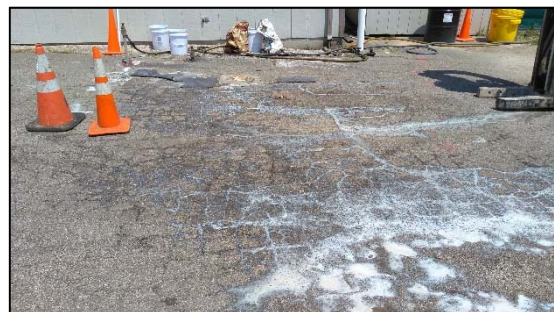
Photo 6: E – Surfacing material through asphalt
