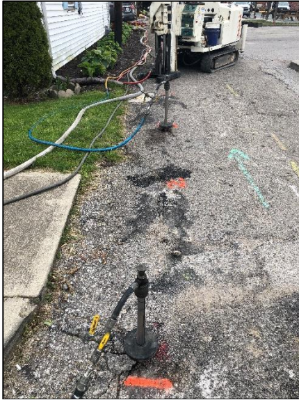
Photo 9: View looking west. Injection equipment and drill rig in view. (May 13, 2020).
