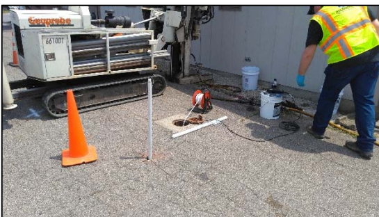
Photo 5: NE – Injecting on IP-1 and monitoring MW-1 and PZ-1
