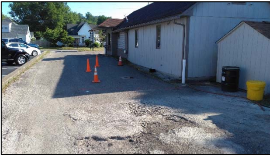
Photo 1: N – MW-1 Injection work area
