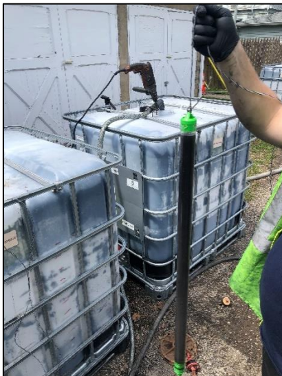
Photo 3: View looking northwest. Bailer drawn from MW-24 showing influence of PlumeStop. (Apr 27, 2020).
