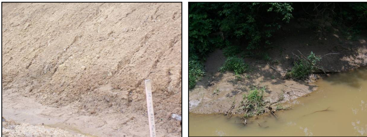
Figures 5.2.2-2 Exposed soil susceptible to runoff and exposed stream banks
