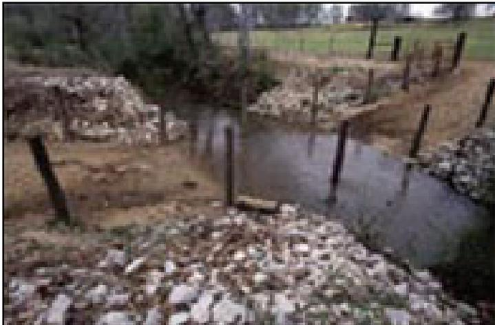
**Plate 8.2** Pictured to the left is an example of “limited access fencing” with a stream crossing, which reduces livestock time in the stream, erosion, and pollution. The sides of these banks were stabilized using rip rap.
