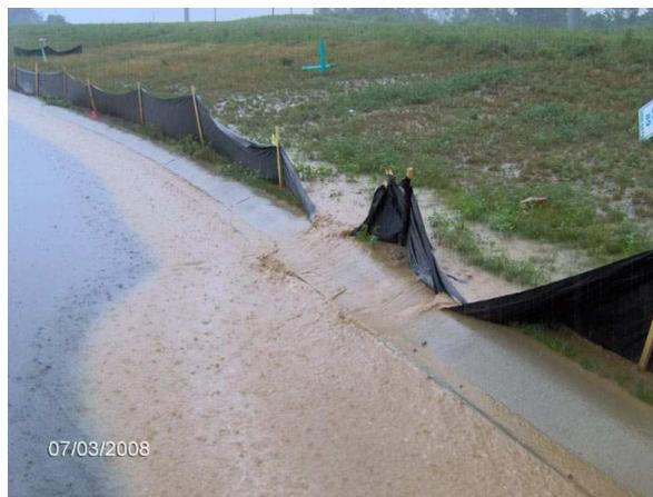
**Figure 4-1: Poorly installed silt fencing**
