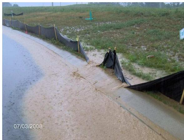
**Figure 4-1: Poorly installed silt fencing**
