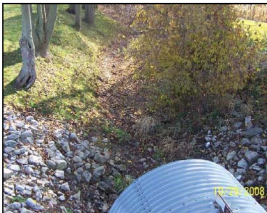
Example of Rip-Rap Stabilized Streambank
