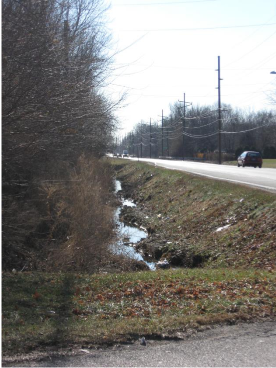
Plate 22: Franklin Road Ditch
