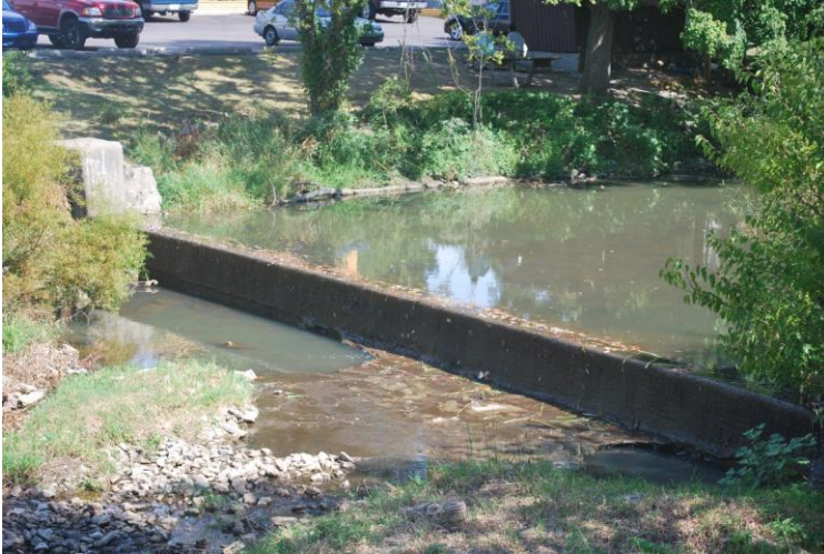
Plate 10: 'Shirley Lake' Dam and Shelby Street Dam
