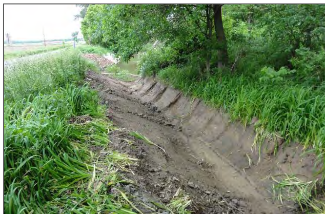
Figure 5 - Ditch Maintenance, Sullivan County
