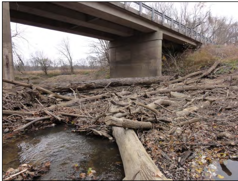
Figure 19 - Log Jam – Dodds 2 Monitoring Site (November 2014)
