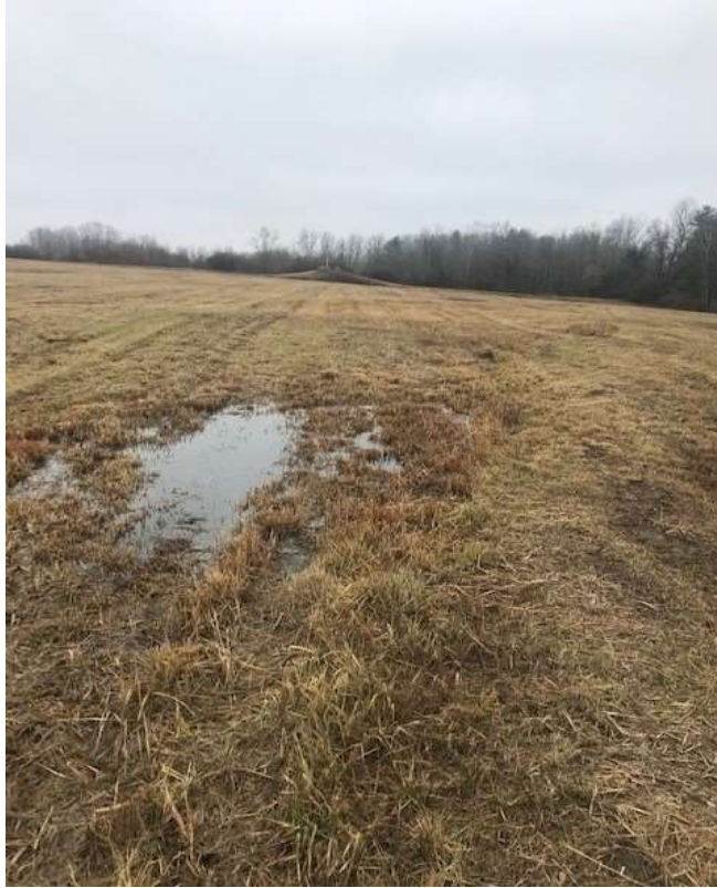
7. View to South Along Landfill Lower Terrace (Minor Ponding)
