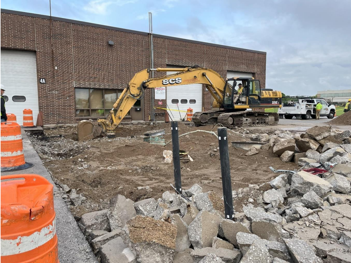
Exposing Tanks (typical)
