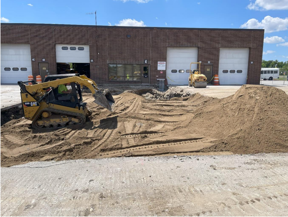
Backfilling Excavation (typical)
