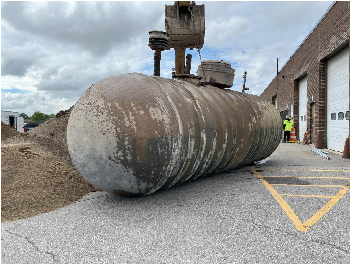
Tank Removal (typical)
