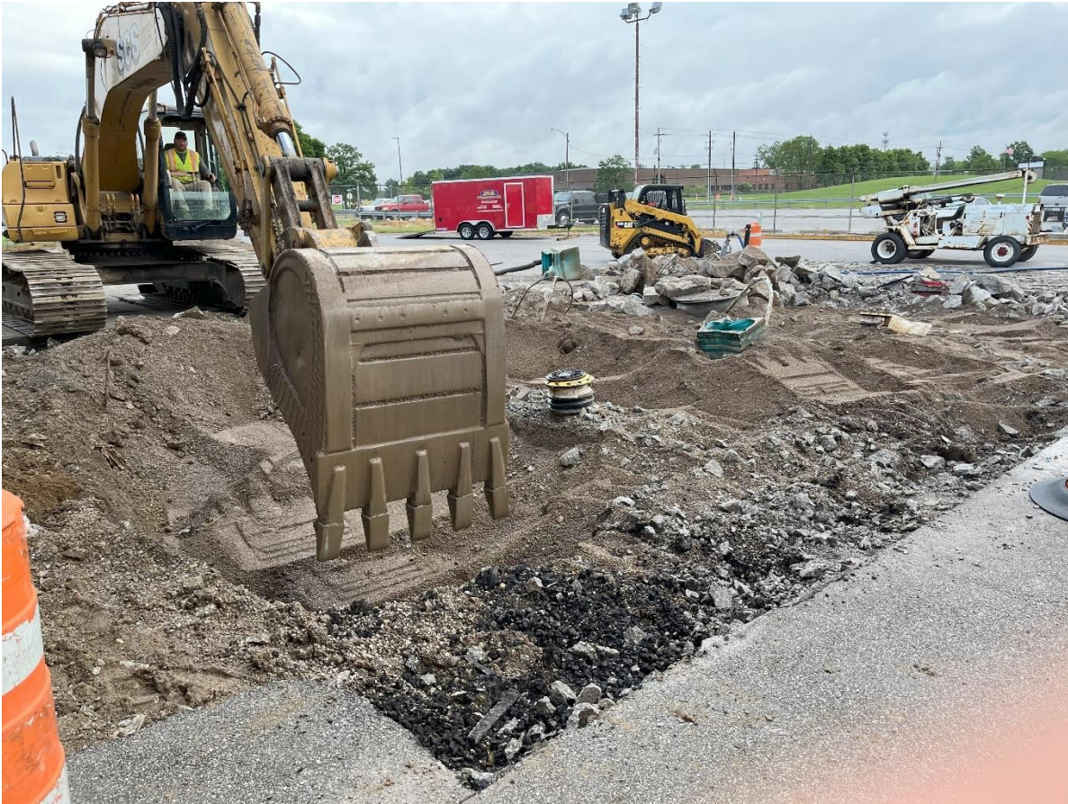
Exposing Tanks (typical)
