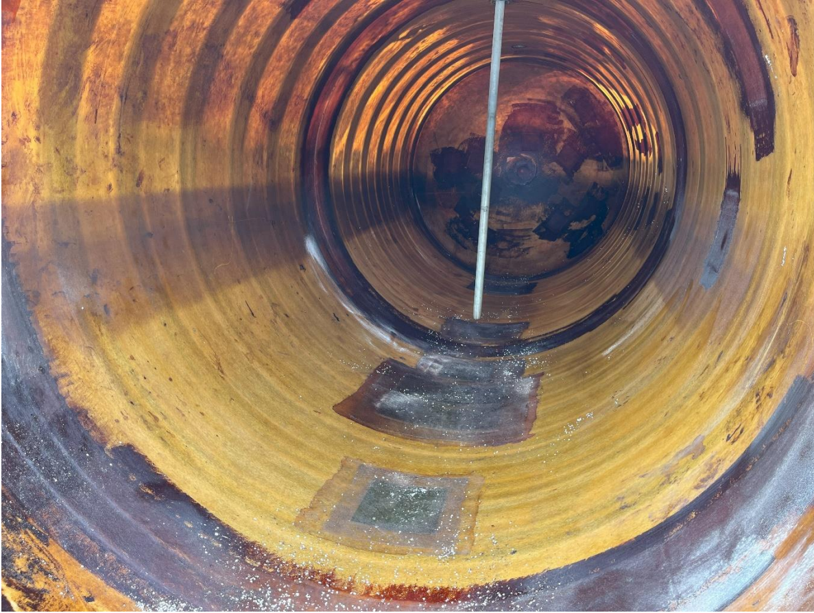
Tank Cleaning (typical view following cleaning)
