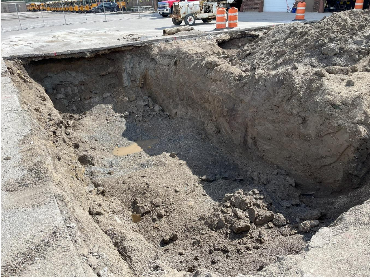
Tank Basin – Excavation Area (typical)
