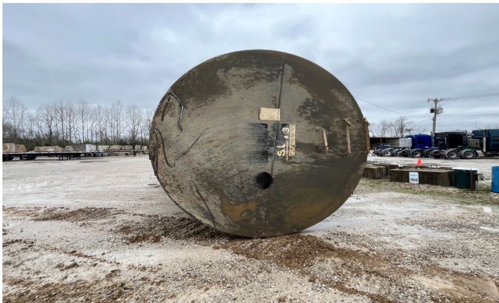
Photo 2 – 15,000-Gallon UST post excavation
