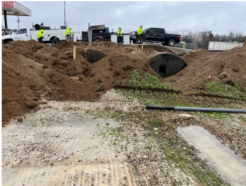
Photo 5 – Photo of both USTs before removal (facing from the west)
