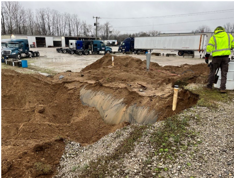
Photo 6 – Photo of both USTs before removal (facing from the southeast)
