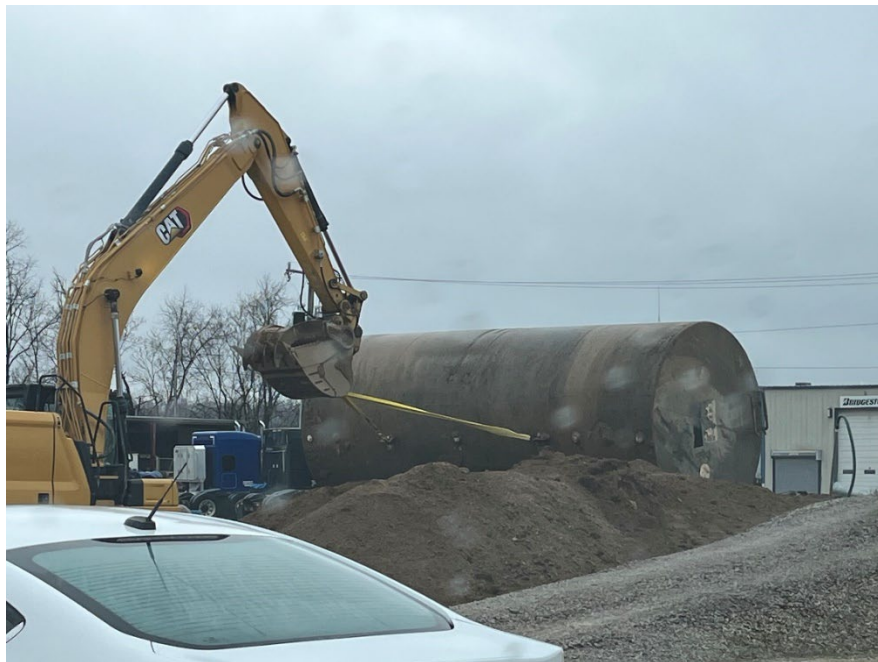
Photo 4 – Photo of the 2 nd UST during removal
