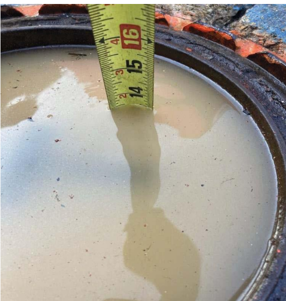
RUL VAPOR REC SPILL BUCKET TEST START 13.5"
