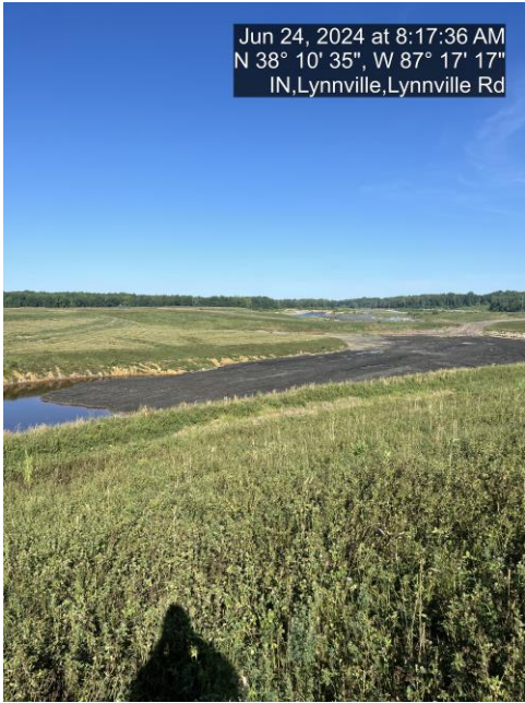
RB010A overview and grading progress.
