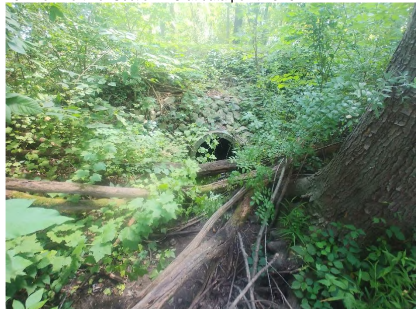
20. View south towards culvert under Midland Trace Trail.
