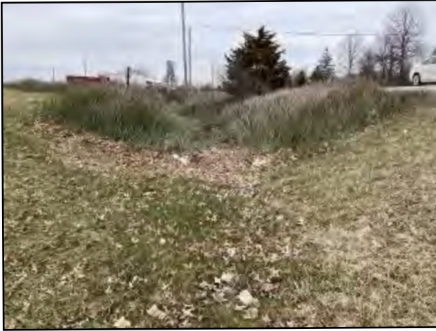
PP14, Looking north (3/21/23)
