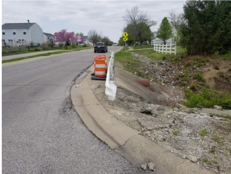
View: Apryl Drive, facing west. Description: Existing bridge over Tracy Ditch.
