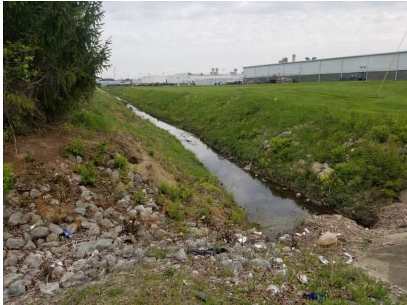
View: Tracy Ditch, facing north. Description: Tracy Ditch north of the bridge.
