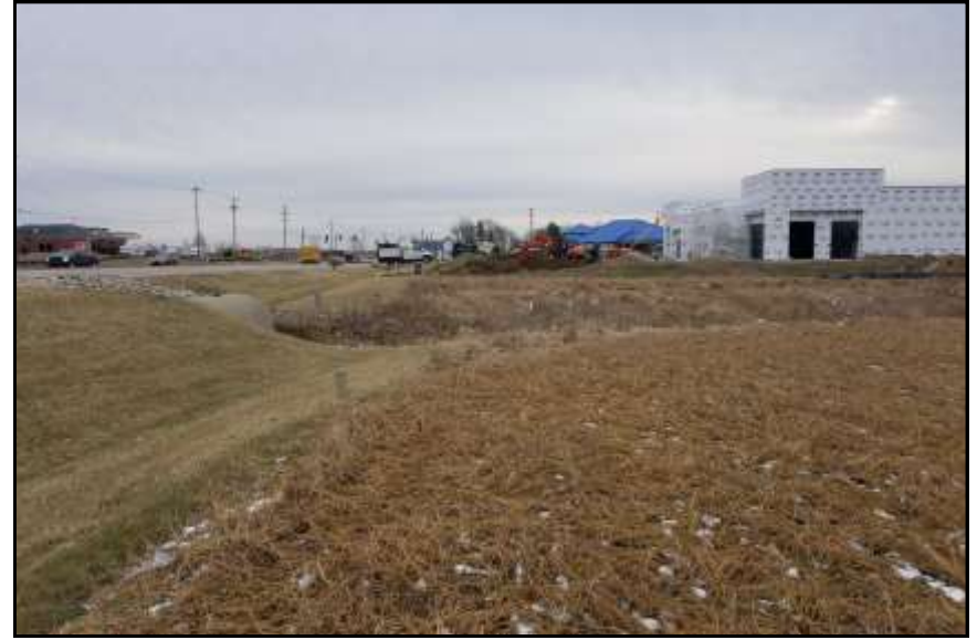
Photo Station 02. View Looking East, 02/14/2019
