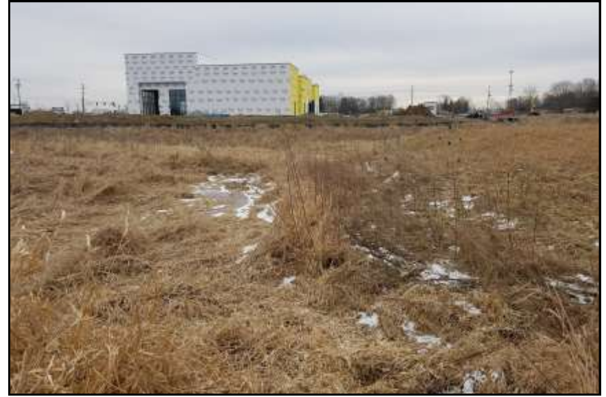
Data Point 2. View Looking East, 02/14/2019
