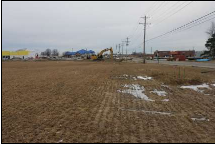
Photo Station 01. View Looking North, 02/14/2019
