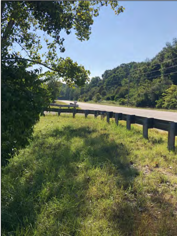
Picture 53—SR 26 roadside northeast quadrant and drive; southeast view; 1 SEP 2021.
