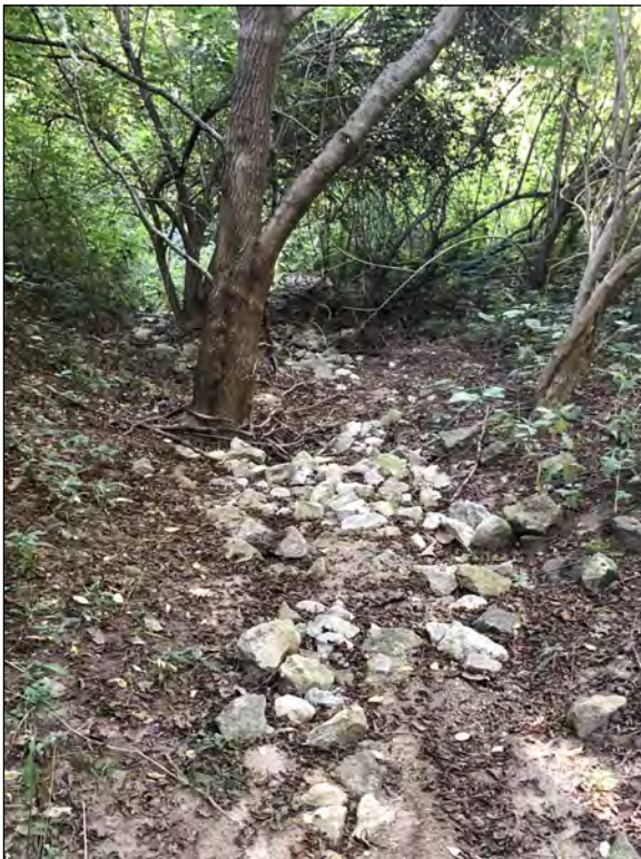
Picture 35—UNT 3 to Goose Creek downstream from end of bed and bank structure—note riprap; east view; 1 SEP 2021.
