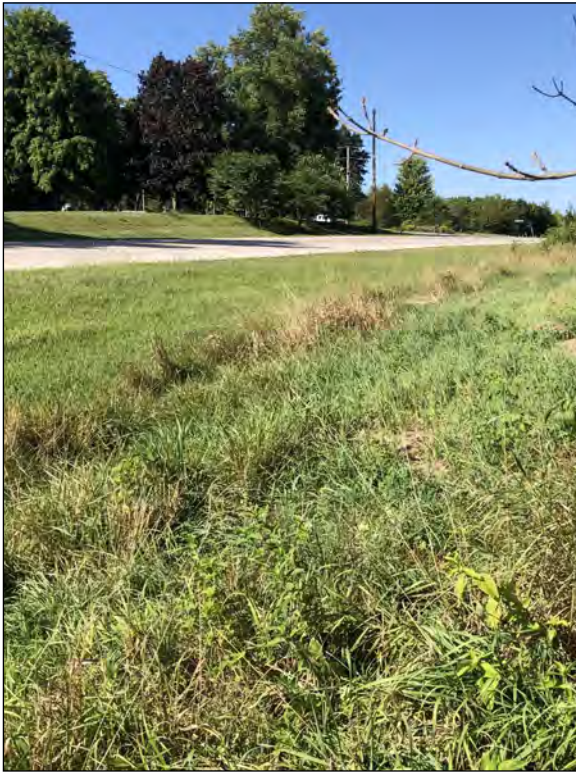
Picture 47—SR 26 roadside from RSD1 end ; southwest view; 1 SEP 2021.
