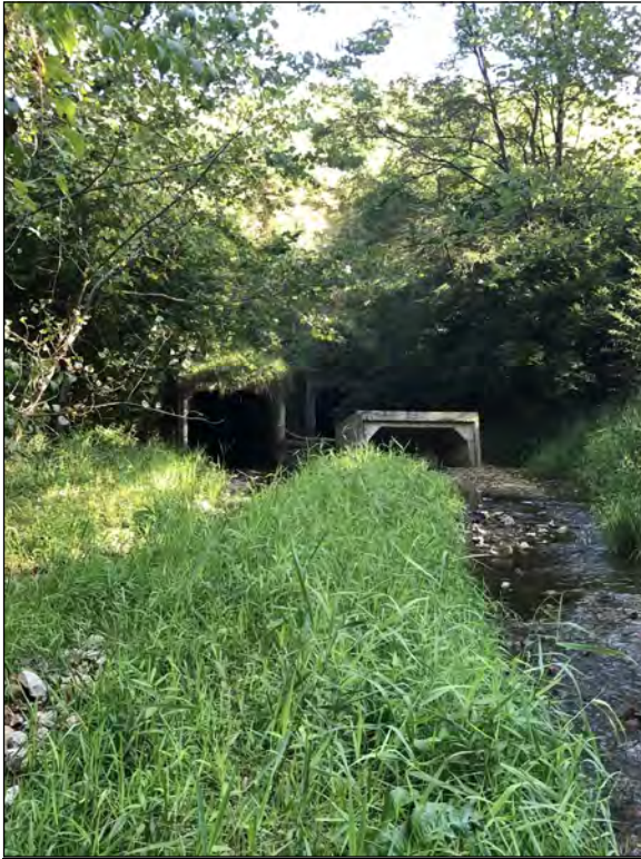
Picture 5—Goose Creek upstream and project structure CV 026-079-28.10 ; north view; 1 SEP 2021.
