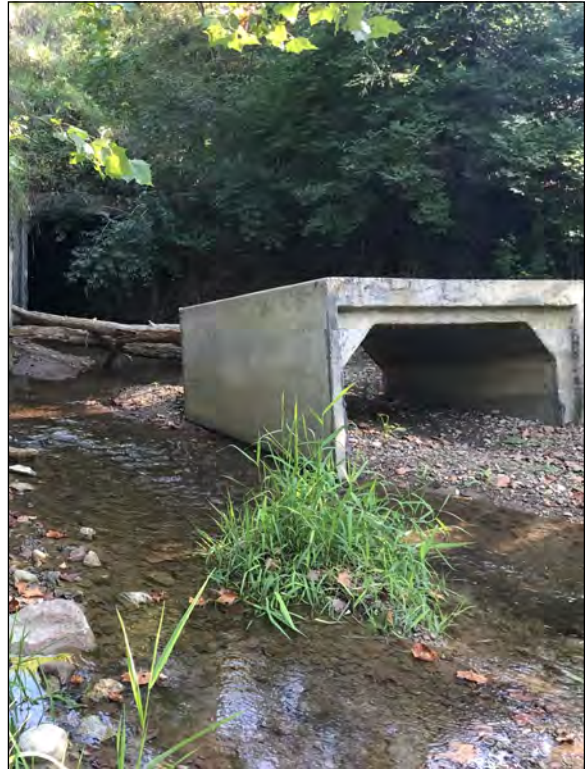
Picture 2— Goose Creek upstream and detached project culvert CV 026-079-28.10 piece; north view; 1 SEP 2021.
