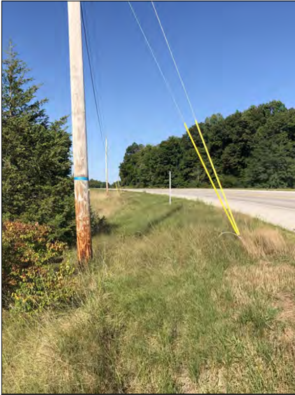
Picture 61—SR 26 roadside southwest quadrant; southwest view; 1 SEP 2021.
