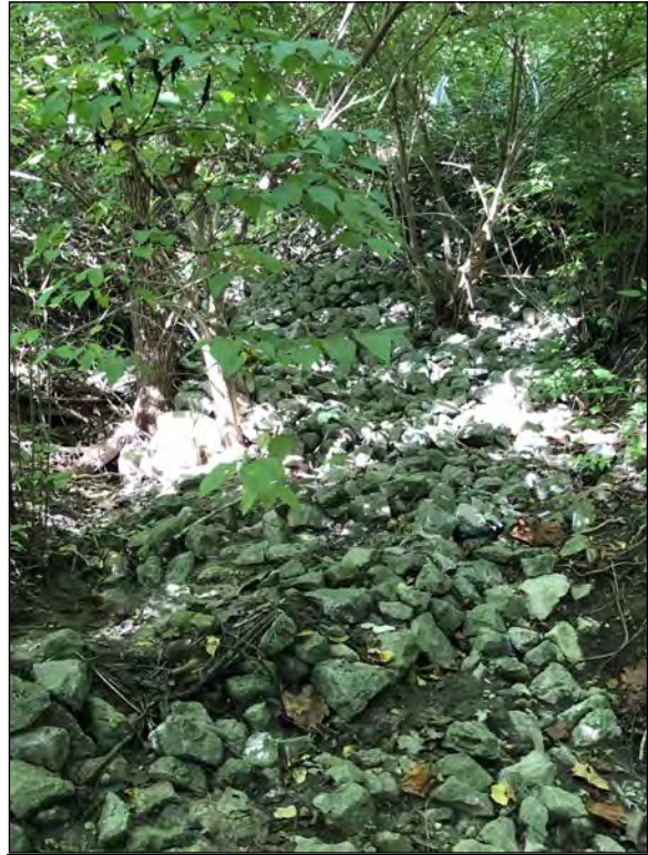
Picture 42—RSD1 riprap area; southwest view; 1 SEP 2021.
