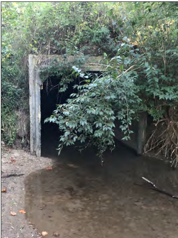
Picture 3—Goose Creek east project structure CV 026-079-28.10 ; north view; 1 SEP 2021.
