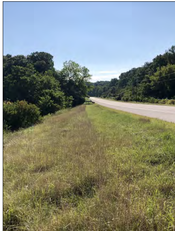
Picture 60—Project center north of SR 26; southeast view; 1 SEP 2021.
