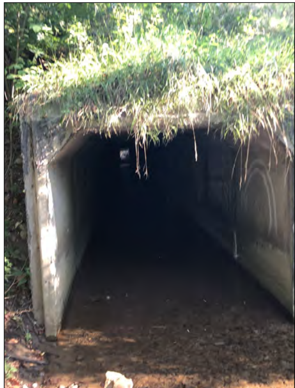
Picture 4—Goose Creek west structure CV 026-079-28.10 ; north view; 1 SEP 2021.
