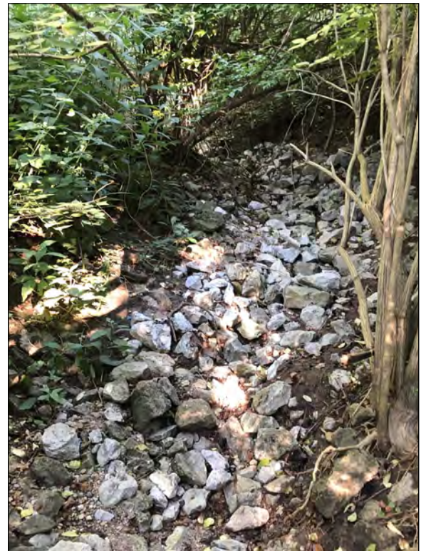
Picture 36—UNT 3 to Goose Creek end of bed and bank structure—note riprap; west view; 1 SEP 2021.
