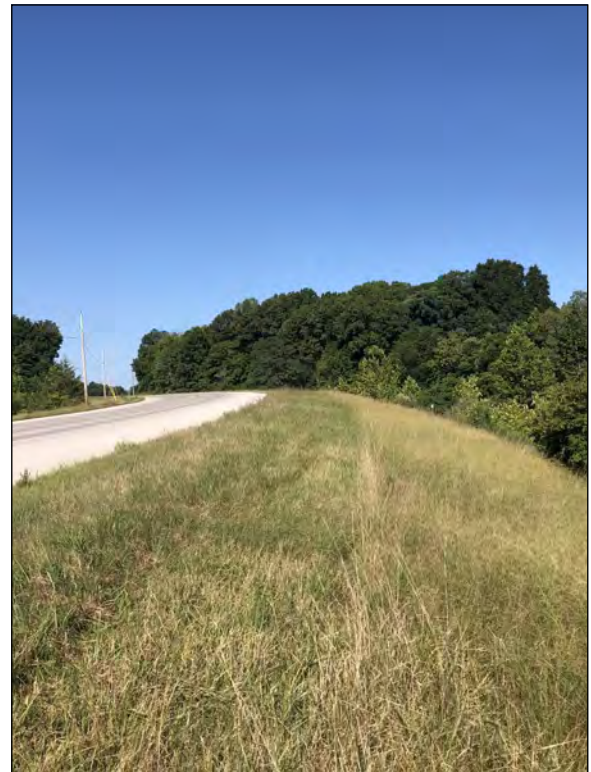
Picture 52—Project center north of SR 26; northwest view; 1 SEP 2021.
