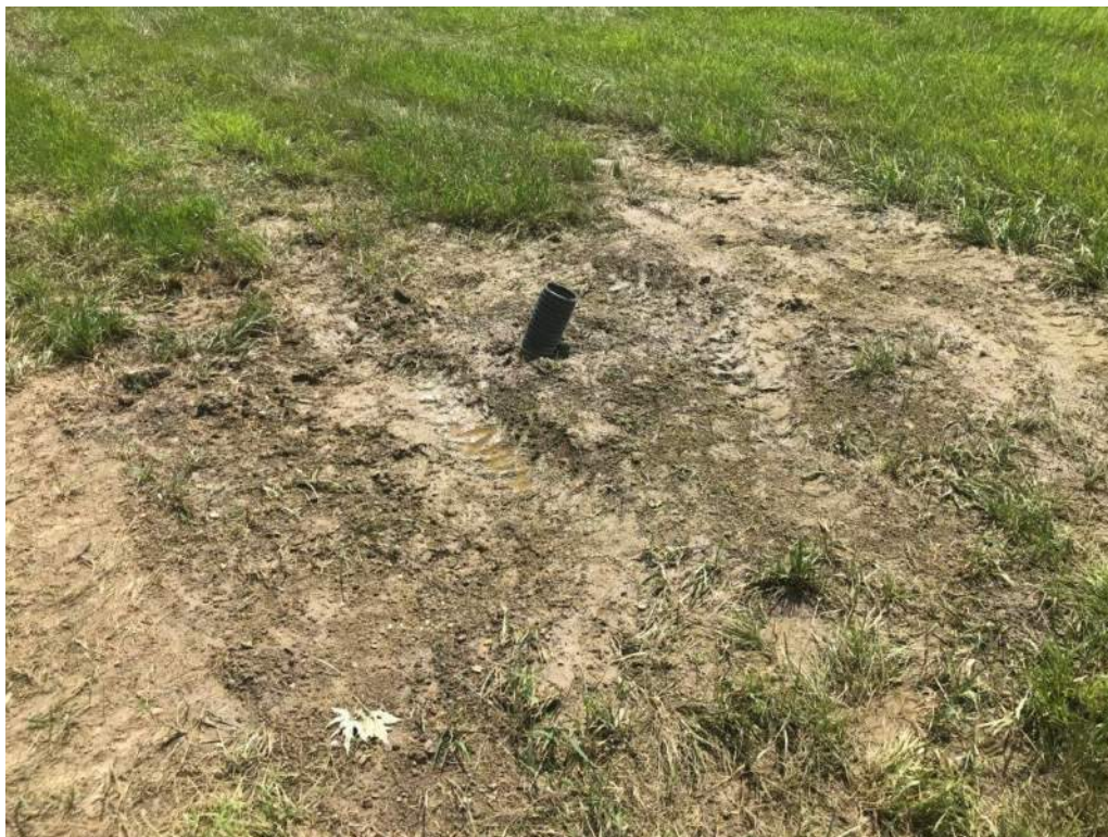
Photo 9: View of tile cleanout area in yard on west side of Proposed Roundabout #1.
