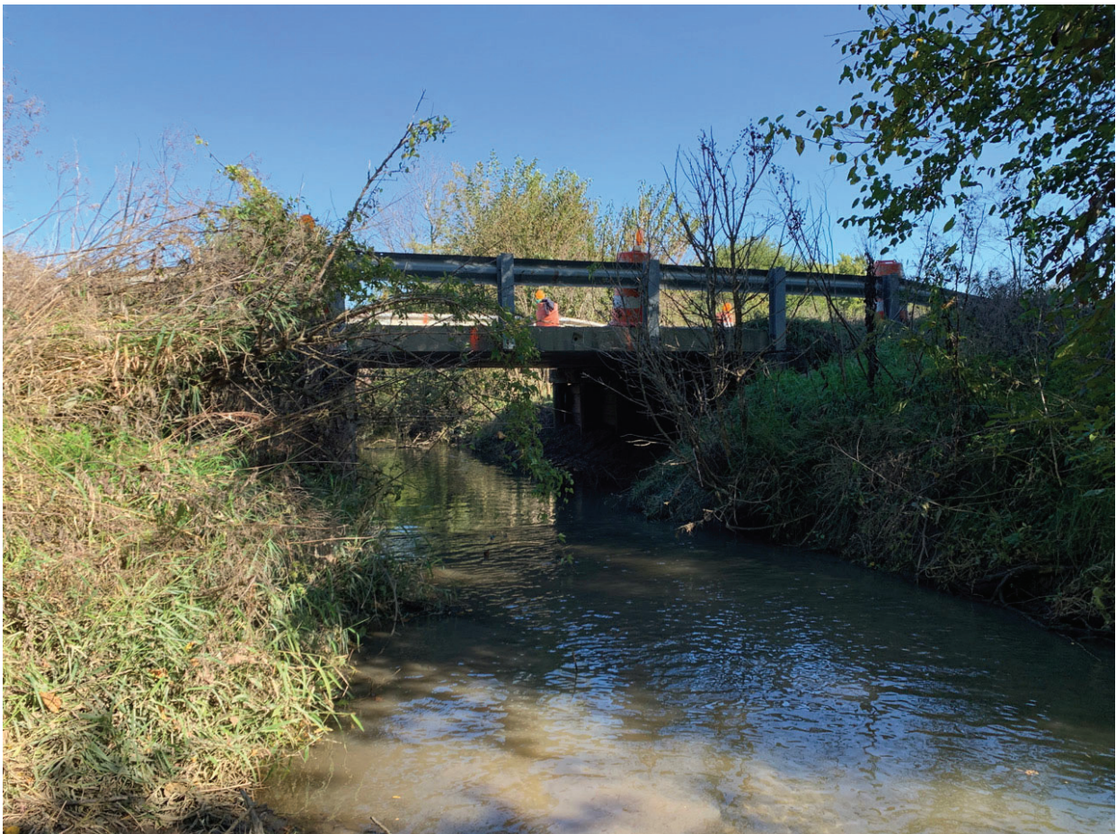
8. Looking northeast upstream along Withe Creek toward structure
