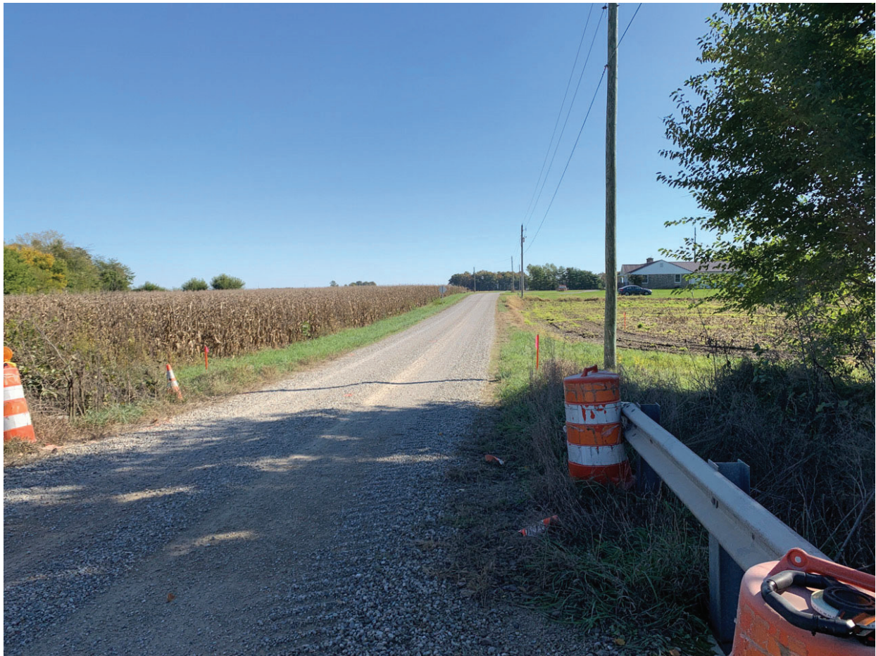
11. Looking east along CR 900 N from structure
