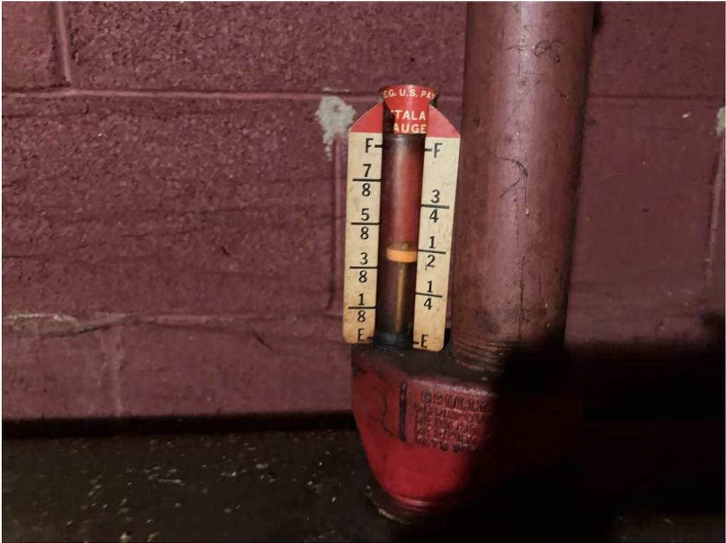
Photo 9: Level gauge on the AST
