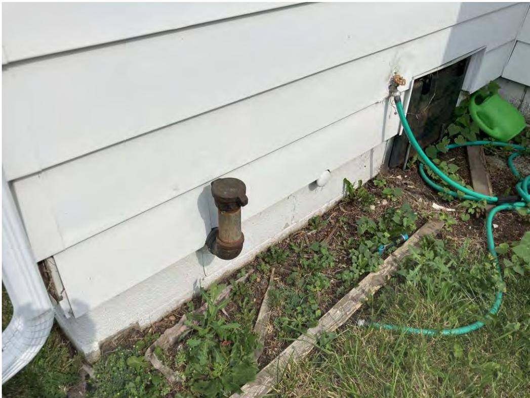
Photo 6: AST fill port and coal door on the south side of the residence
