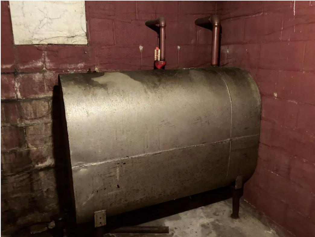
Photo 8: Heating oil AST in the basement
