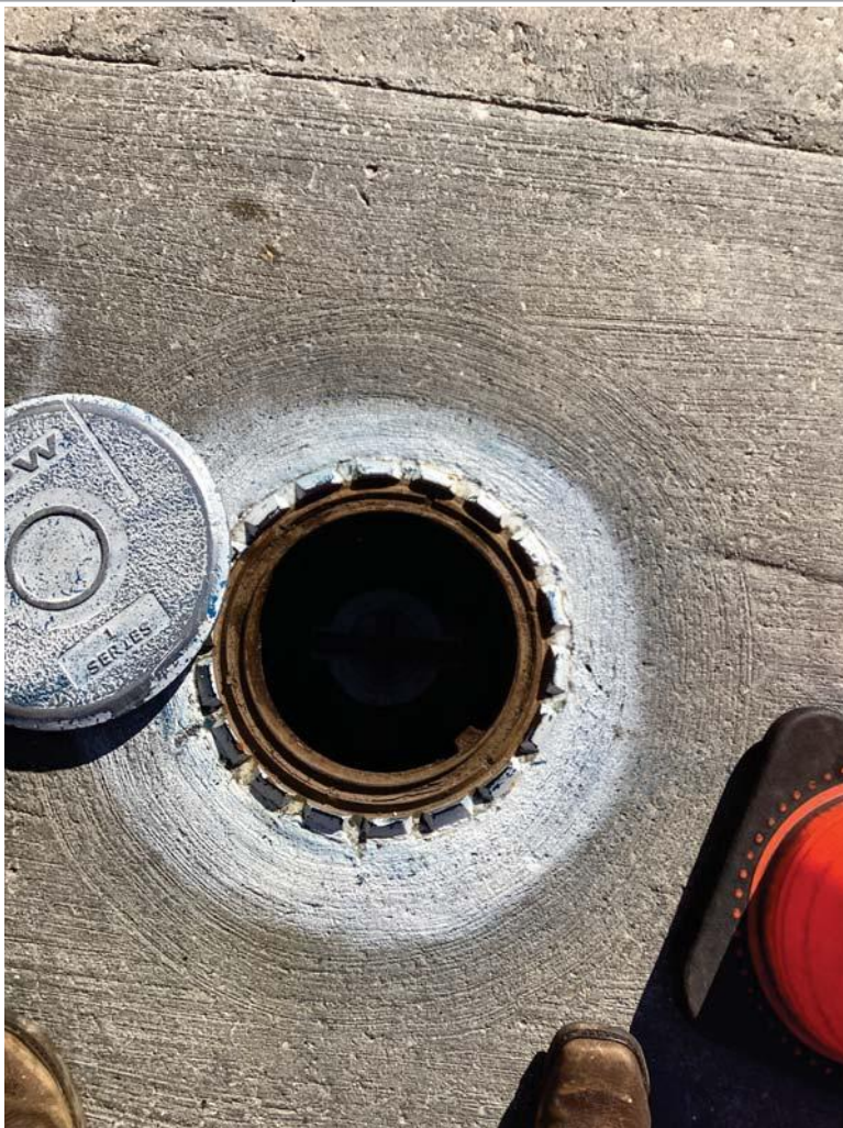
Monthly Inspection Checklist -> Spill Prevention -> Spill Containment Manhole (Spill Buckets) - Free of water and product
