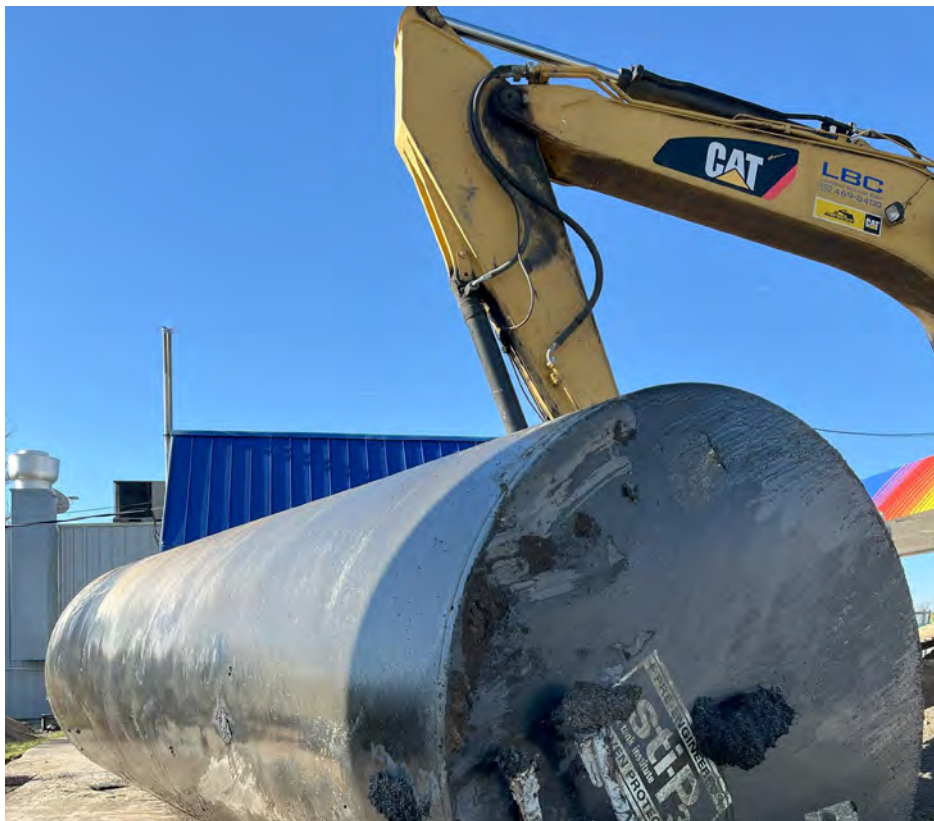
Photo 6: Tanks removed from gasoline basin excavation.
