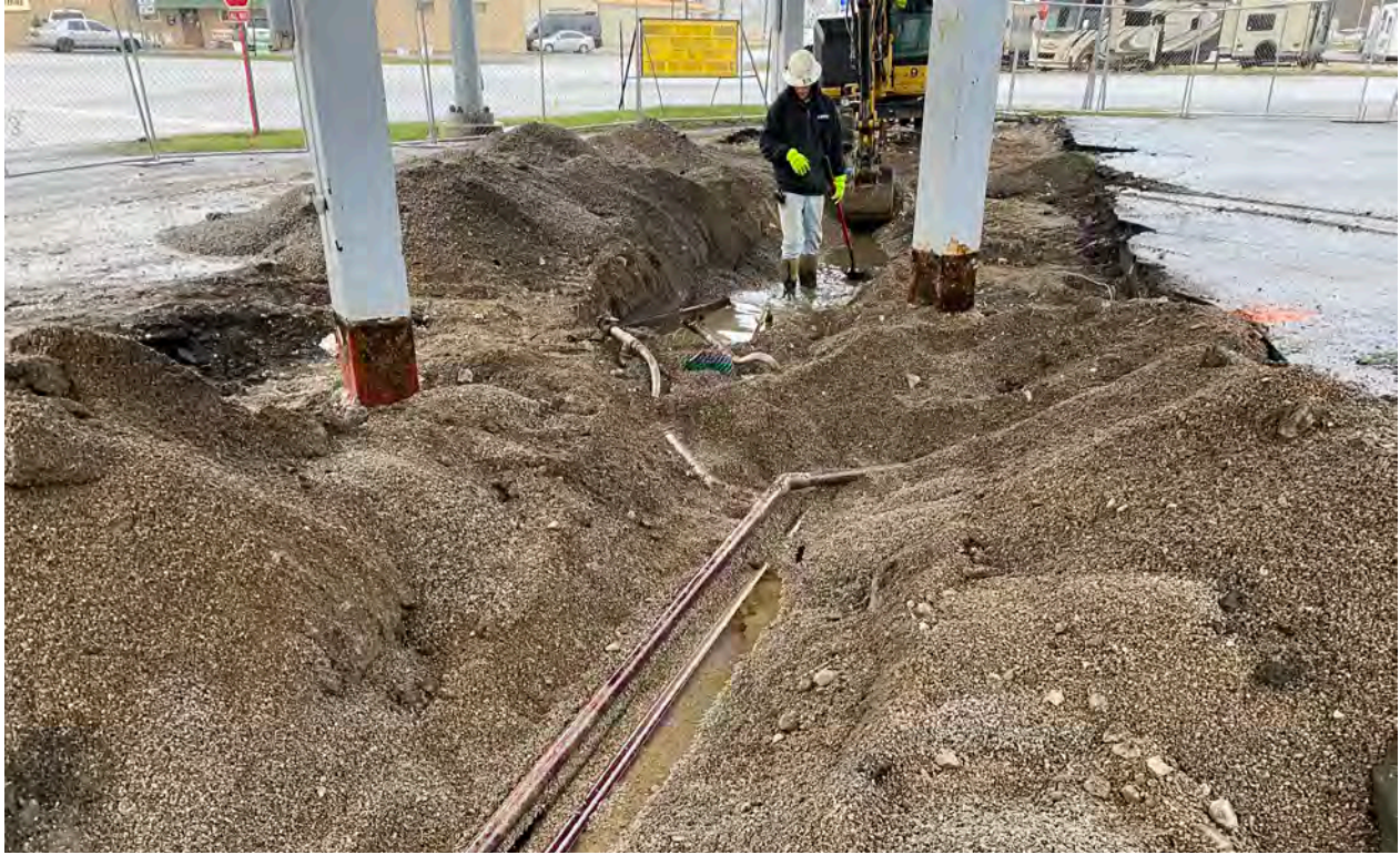
Photo 3: Piping exposed and dispensers removed under fueling canopy.
