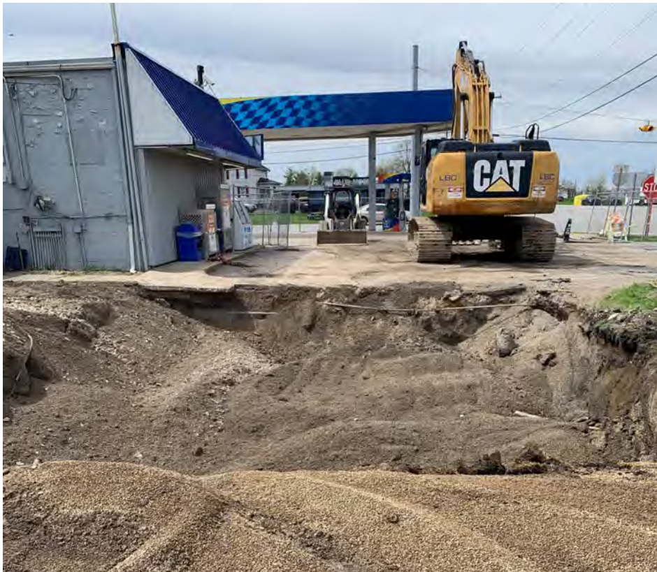
Photo 8: Backfilling of gasoline basin.
