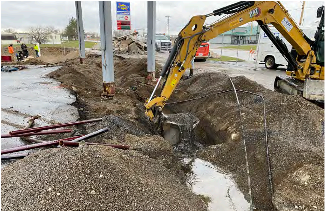
Photo 4: Removing piping under canopy.
