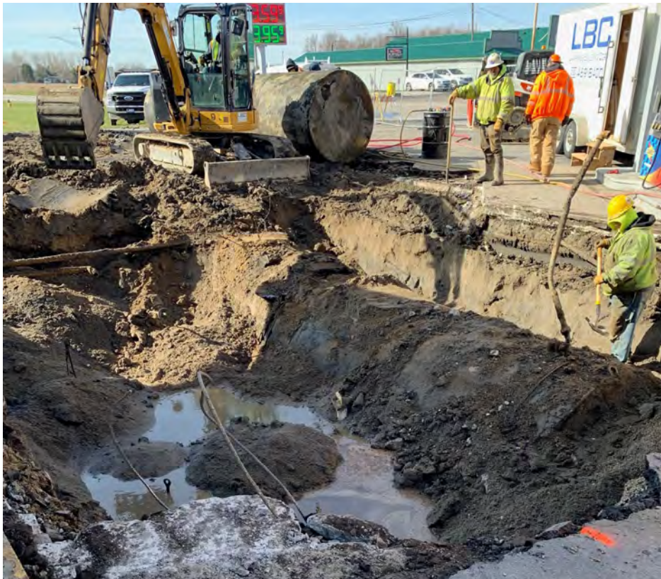
Photo 2: Diesel Tank Basin. Diesel tank removed and exposed orphan tank.
