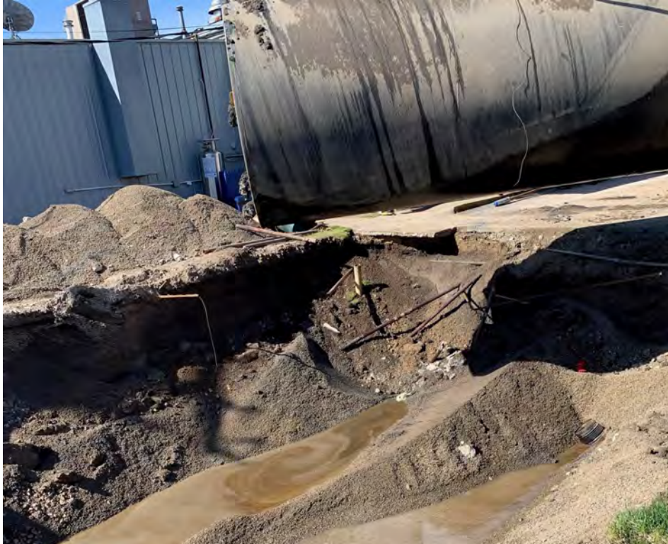
Photo 5: Gasoline basin tank removal. Note sheen on water in excavation.
