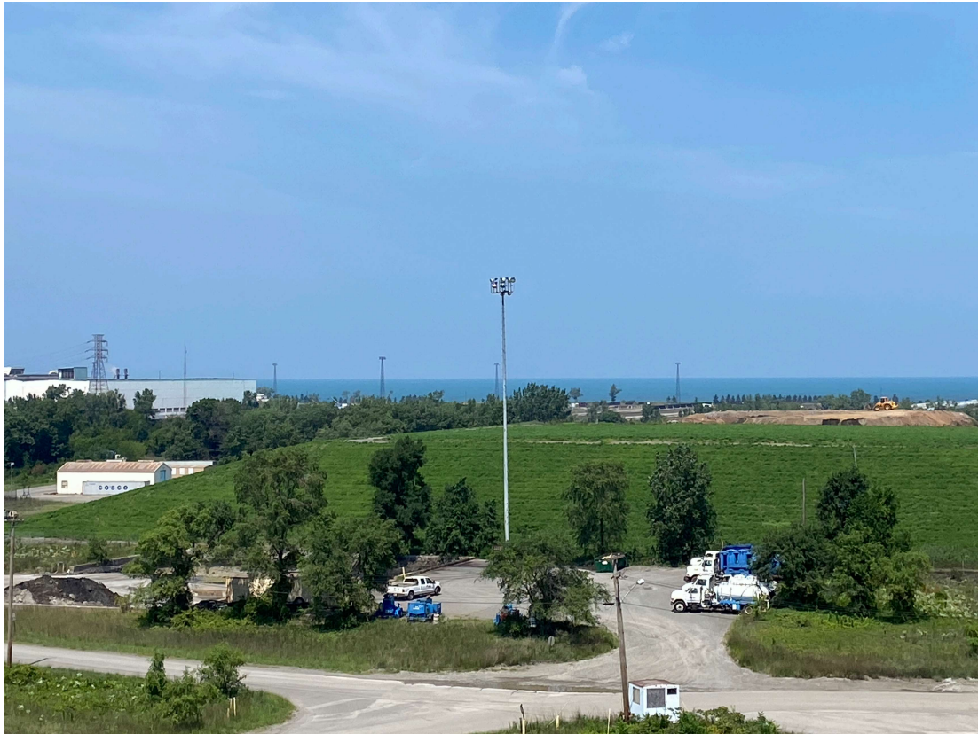
Close up view of Cell B, looking north.
