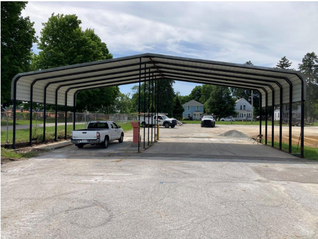
Photo 18. Dispenser area following backfilling
