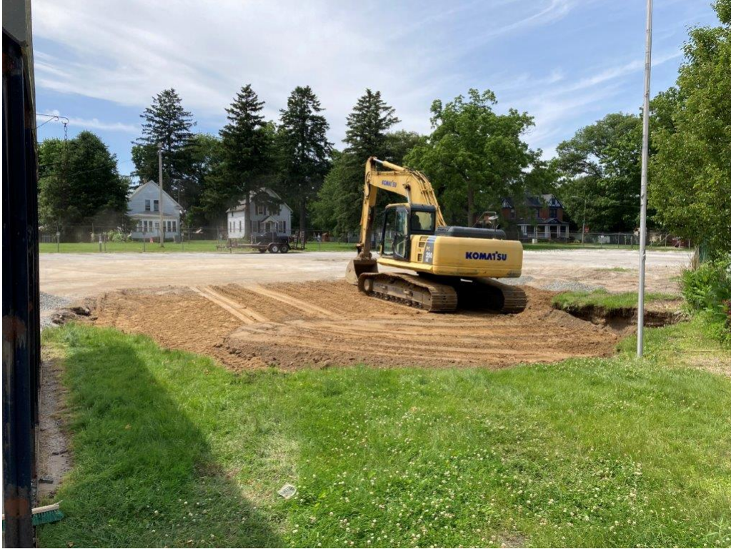
Photo 15. Backfilling excavation
