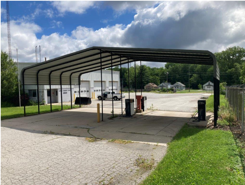
Photo 2. Dispensers prior to removal facing east
