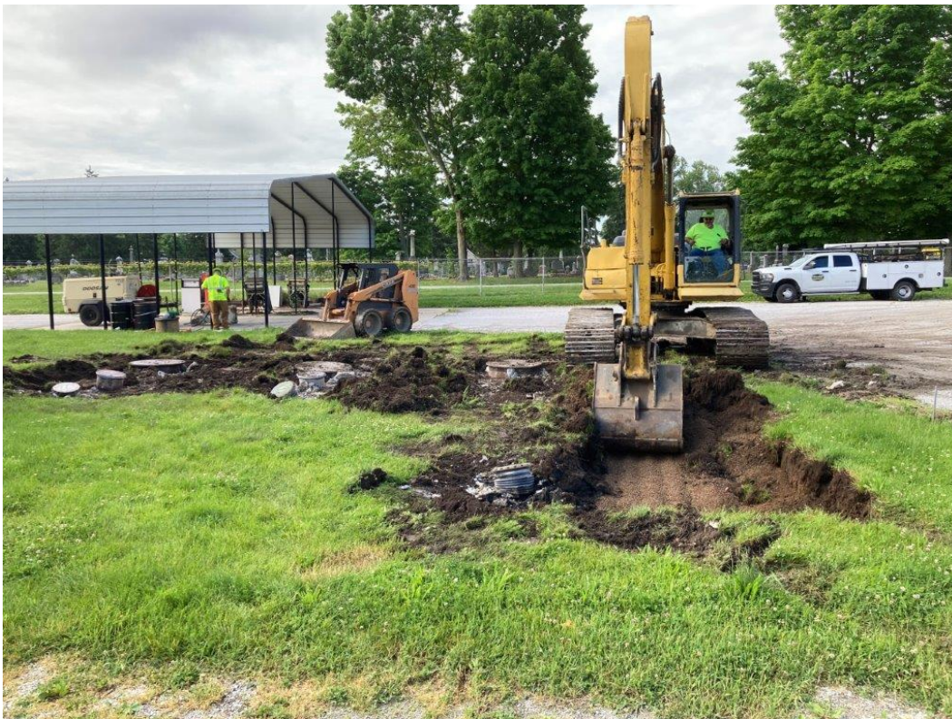
Photo 4. Excavating to top of USTs
