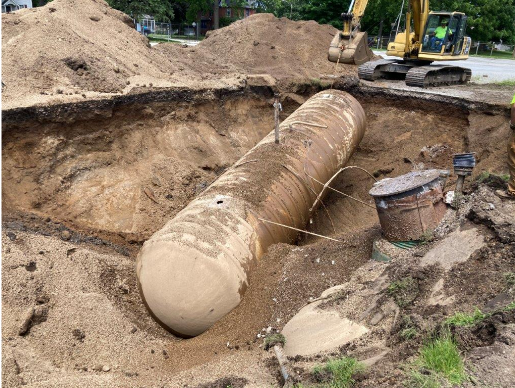
Photo 5. Removing 12,000-gallon diesel UST
