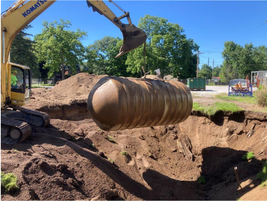
Photo 9. 6,000-gallon gasoline after removal
