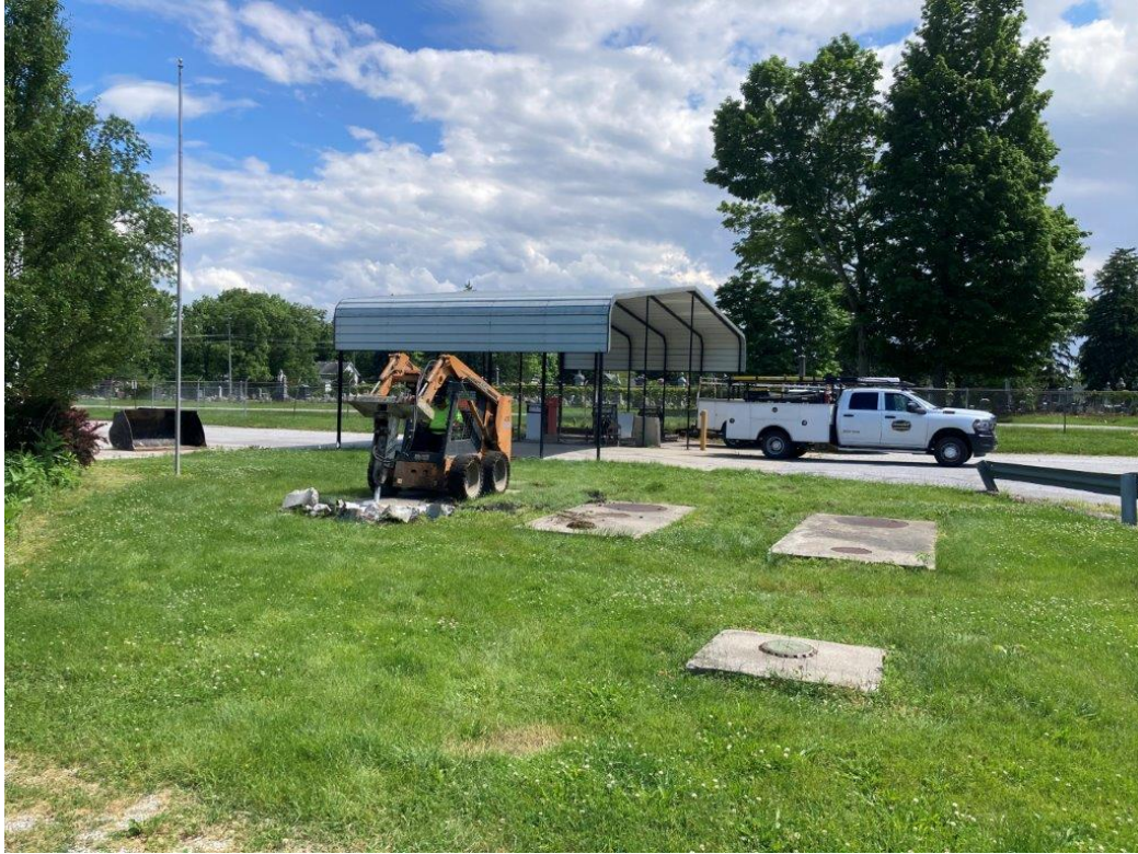
Photo 3. Breaking concrete pad above UST
