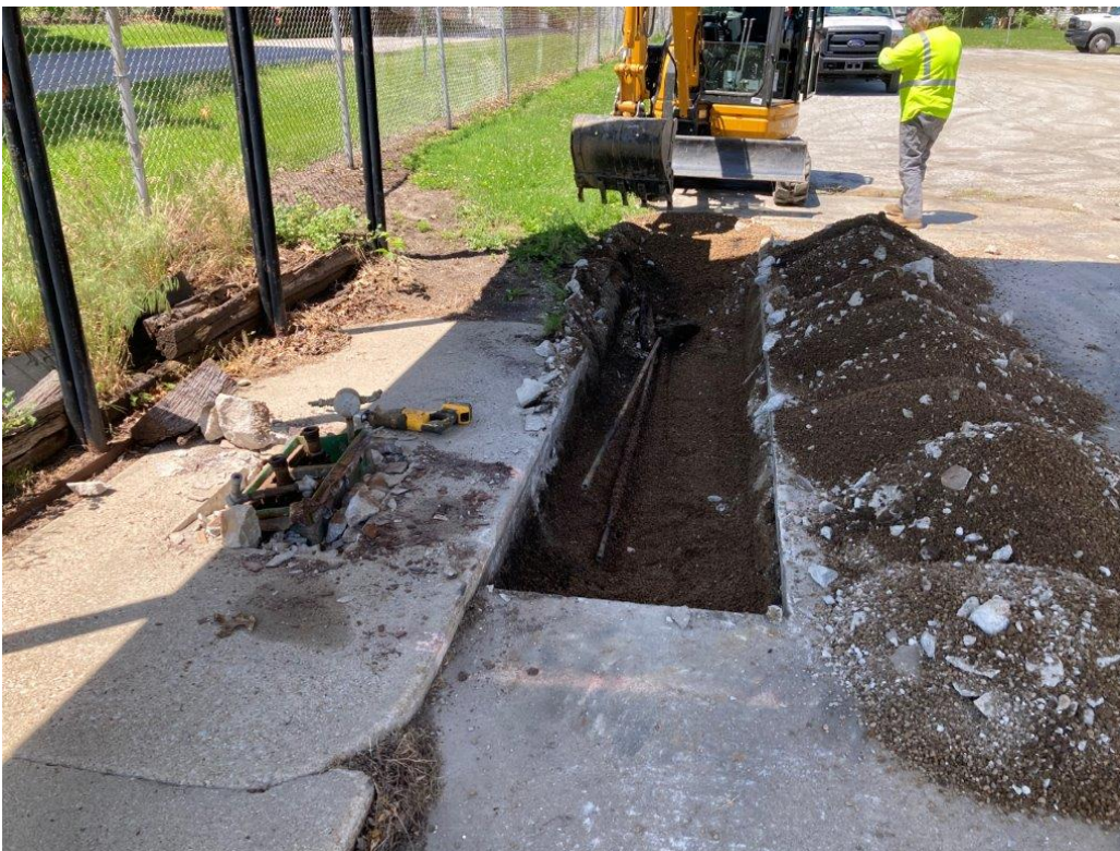
Photo 12. Removal of western product piping
