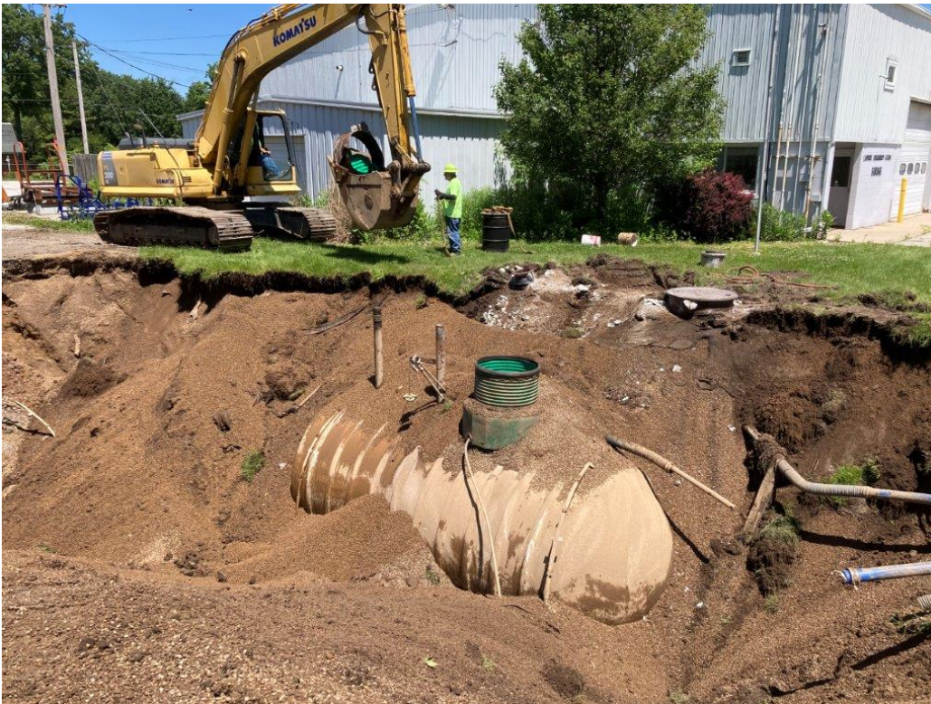
Photo 6. 6,000-gallon diesel UST prior to removal
