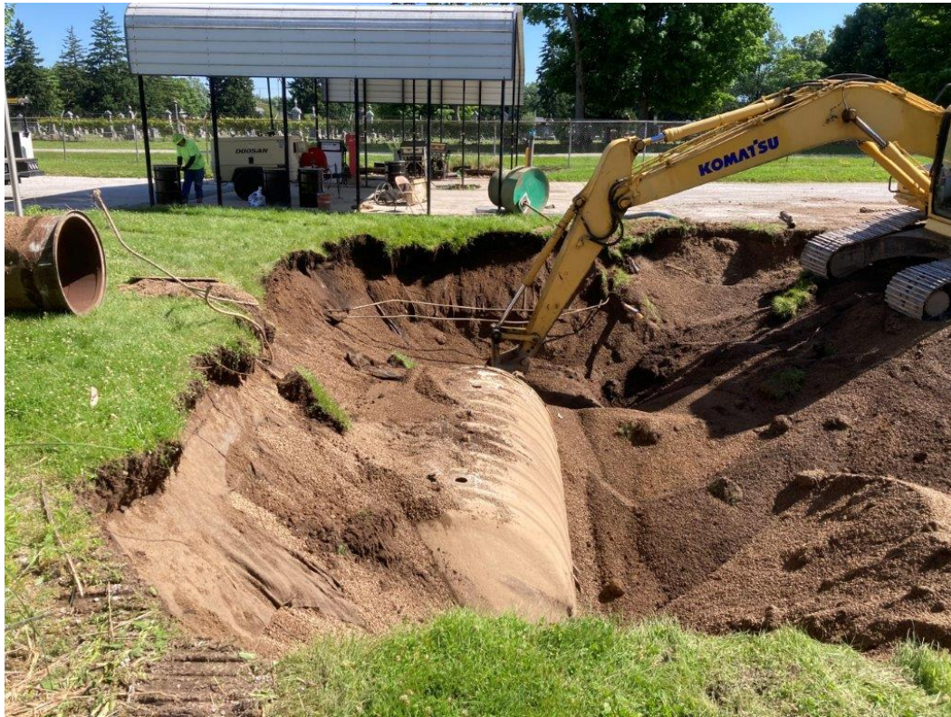
Photo 8. 6,000-gallon gasoline UST before removal
