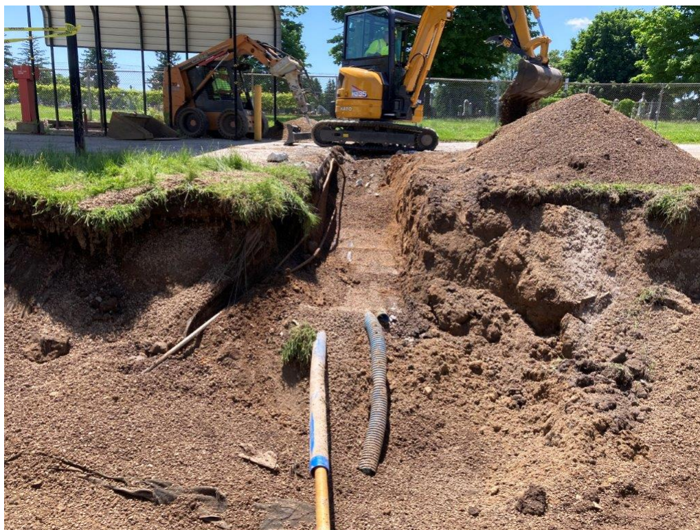
Photo 14. Removal of northern product piping
