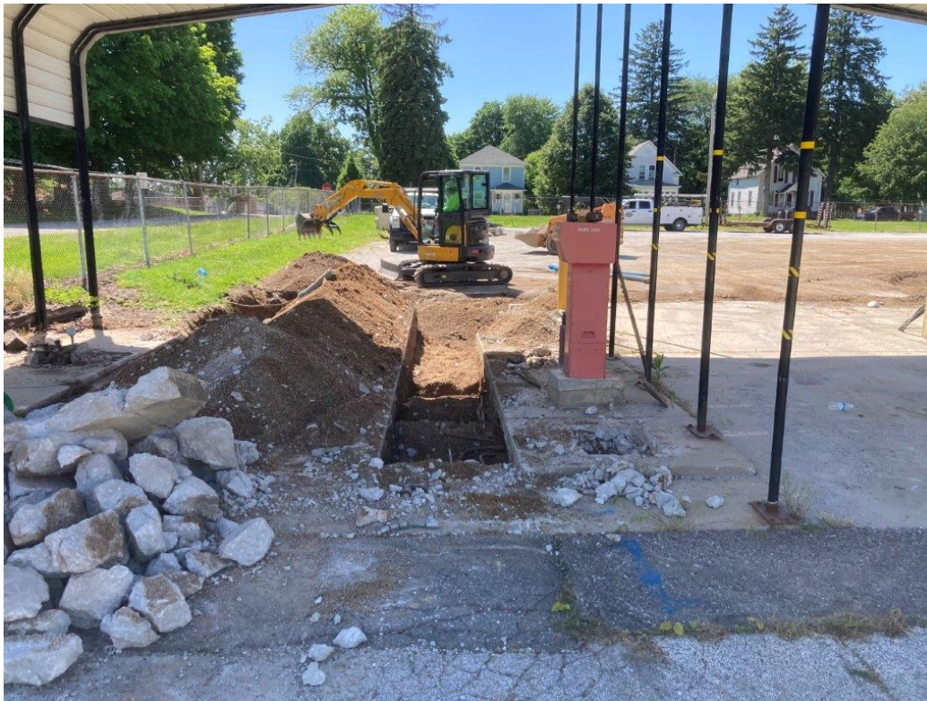
Photo 13. Removal of eastern product piping
