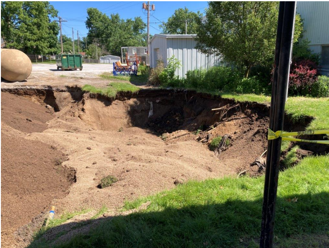
Photo 10. UST basin following UST removal
