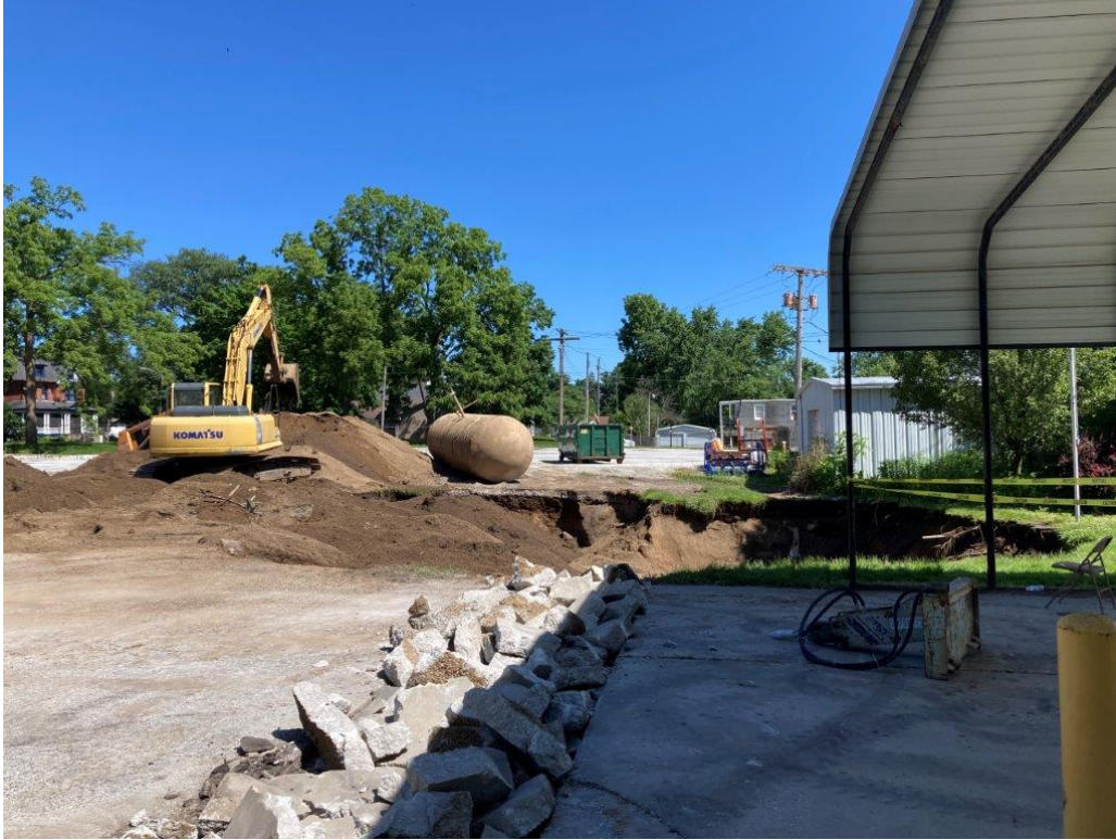
Photo 11. Broken concrete to remove product piping
