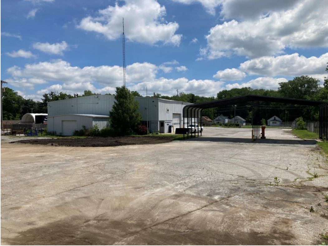
Photo 17. Former UST basin and dispensers following backfilling
