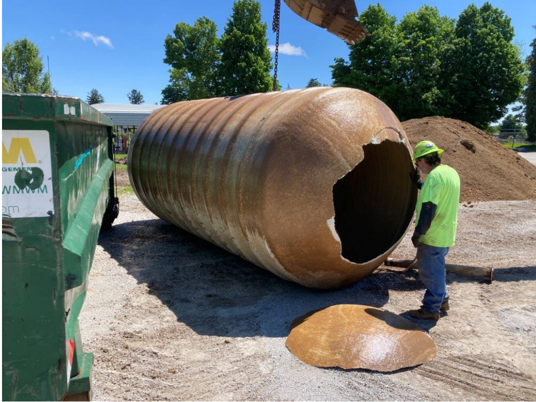
Photo 7. 6,000-gallon diesel UST after removal
