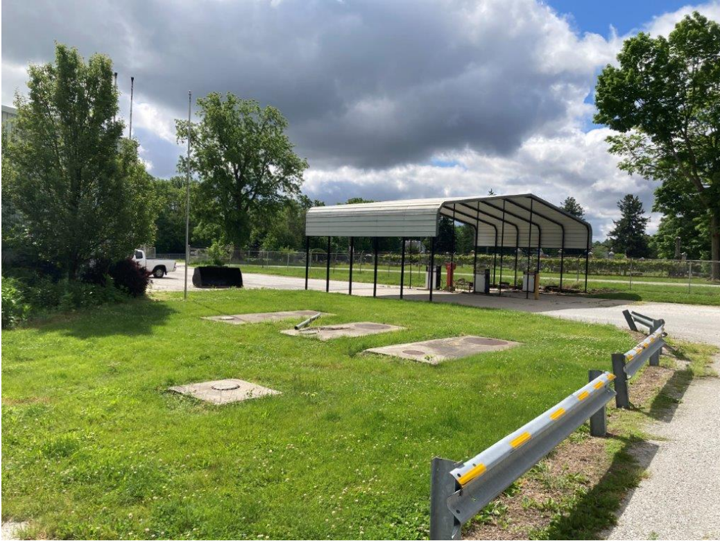
Photo 1. USTs and dispensers prior to removal facing southeast
