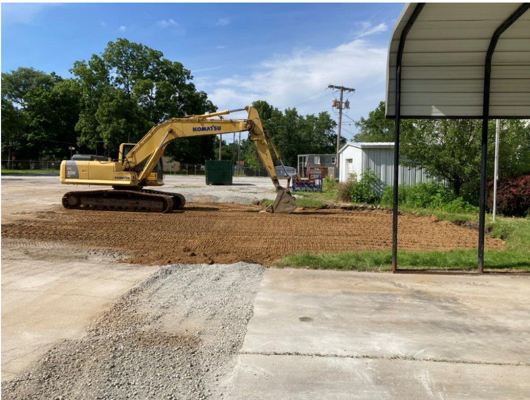
Photo 16. Backfilling excavation
