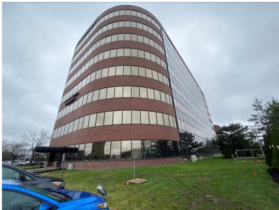
Photo #1: View of site building and UST area (4/6/2022).
