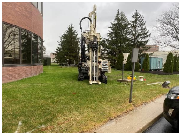
Photo #6: View of soil boring SB-3 (4/6/2022).
