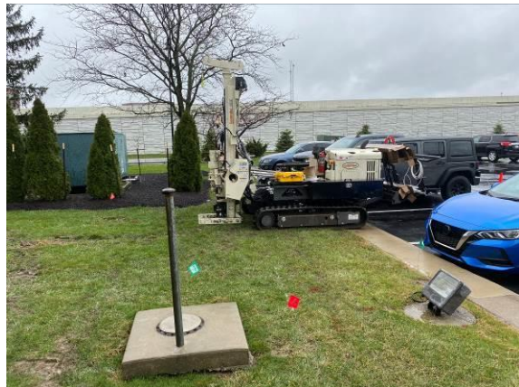
Photo #4: View of soil boring SB-1 (4/6/2022).
