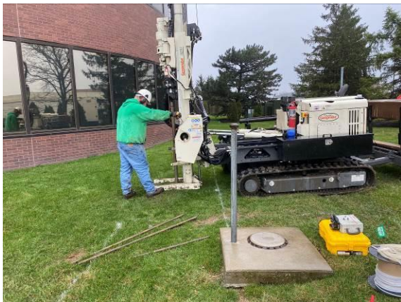
Photo #5: View of soil boring SB-2 (4/6/2022).
