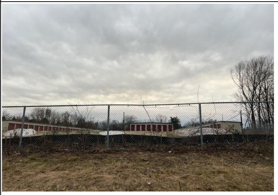
Photo #4 View of fence after Patriot performed repairs.
