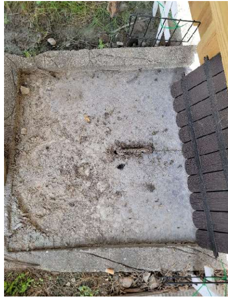
View looking down on the exterior vault.
