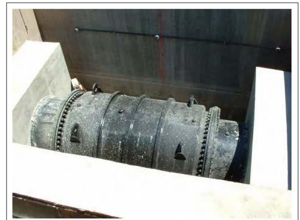
Figure 4-9 72-Inch Pinch Valve
