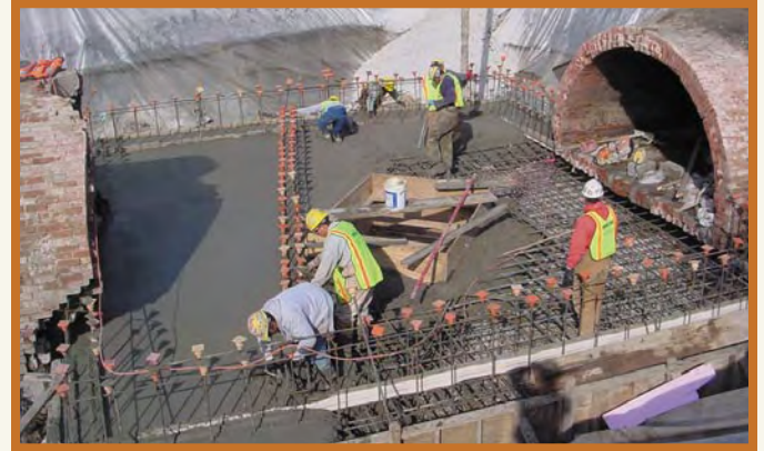
Walsh Construction crew members pour concrete to create a wastewater collection structure under East Michigan Street near Pogues Run. Eventually, three sewer pipes will converge into the underground box, which will direct overflows into an underground tunnel and away from area schools and neighborhoods.
