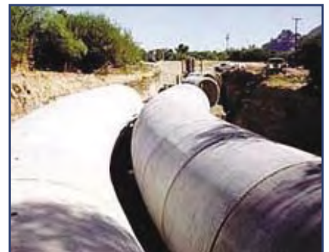
Sewer separation under construction
