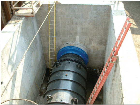
The pinch valve system diverts flows from sewers that overflow during a storm to sewers that aren't full.
