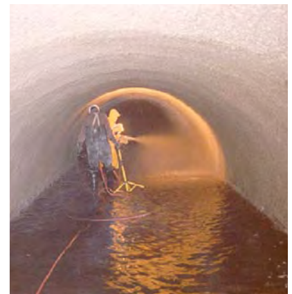
Shotcrete can add life to older sewers at less cost and less disruption than building new sewers.
