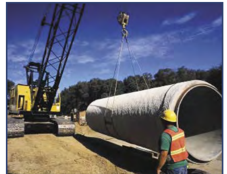
Sewer separation under construction
