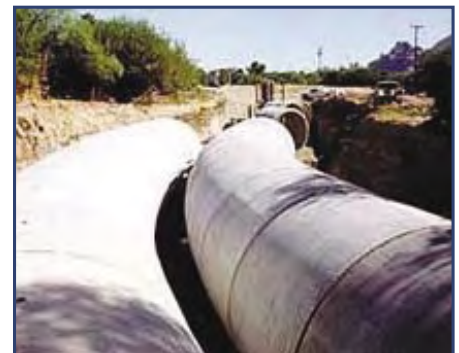
Sewer separation under construction
