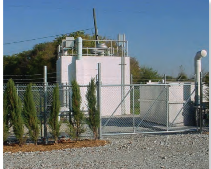
The odor control device (above) helps remove a variety of odors associated with wastewater and sewage. It sits next to a junction chamber that receives wastewater from northeastside neighborhoods.
