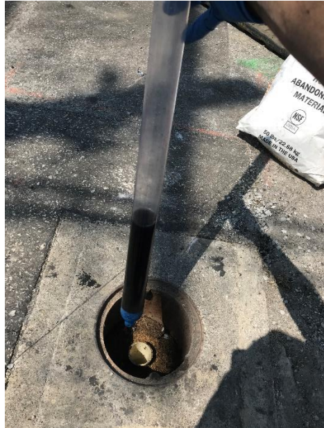
Photo 6: View looking north. Post-injection picture of bailer at MW-10 showing jet black color, indicating strong influence. (August 2, 2018)
