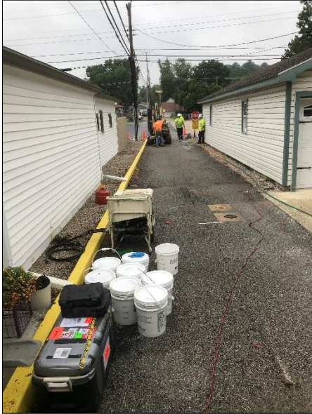
Photo 1: View looking north. BDI cooler, HRC buckets, GeoProbe GP300 Grout Pump, Drill rig, Midway and RRS personnel in view. (July 30, 2018)
