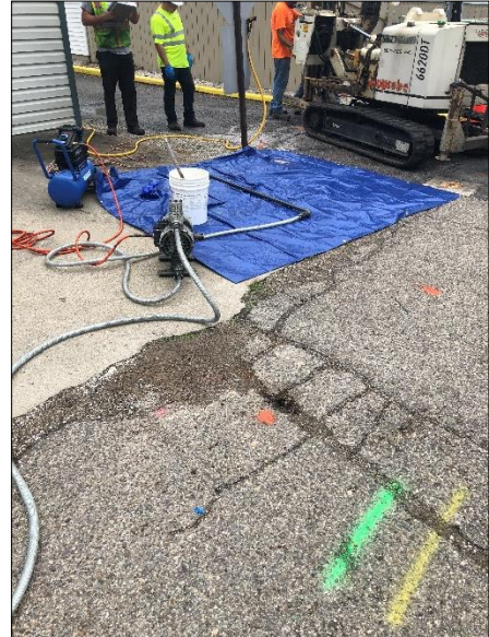
Photo 4: View looking southeast. RRS personnel in view injecting HRC with a Yamada pump. (July 30, 2018)
