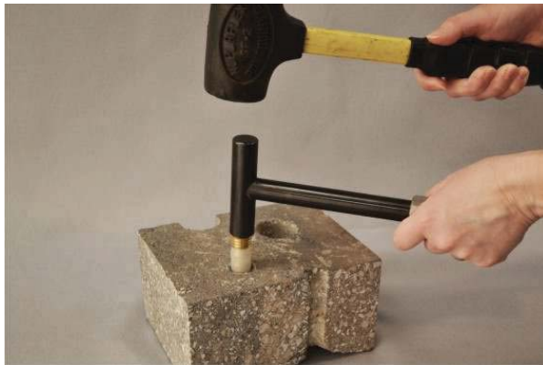
Figure 2. Installing the Vapor Pin™.
