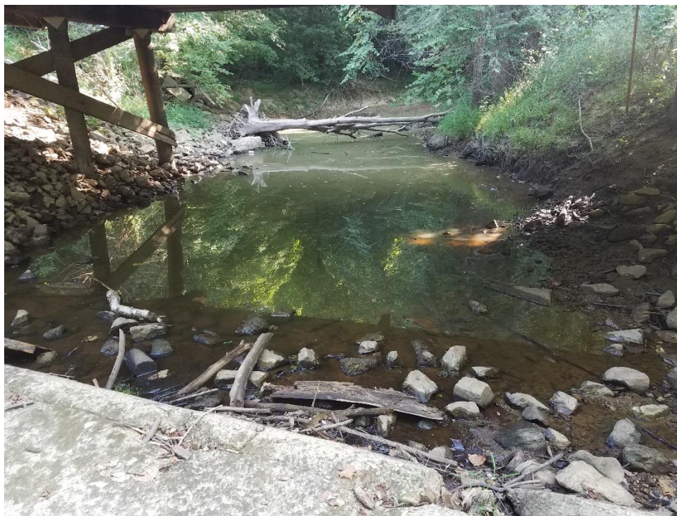
Figure 60: Structure at site WEL170-0008 showing movement of stream at upstream portion. Buildup of debris further prevented water movement by blocking drainage pipes under structure.
