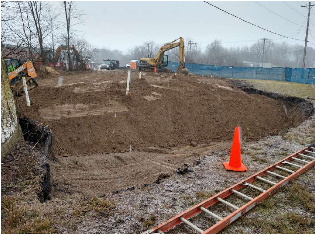
Photo 19: Continued backfill of excavation area (February 26)
