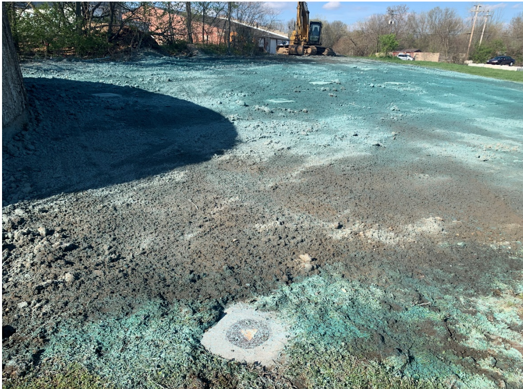
Photo 23: Final grade with hydroseed looking northeast (April 10)
