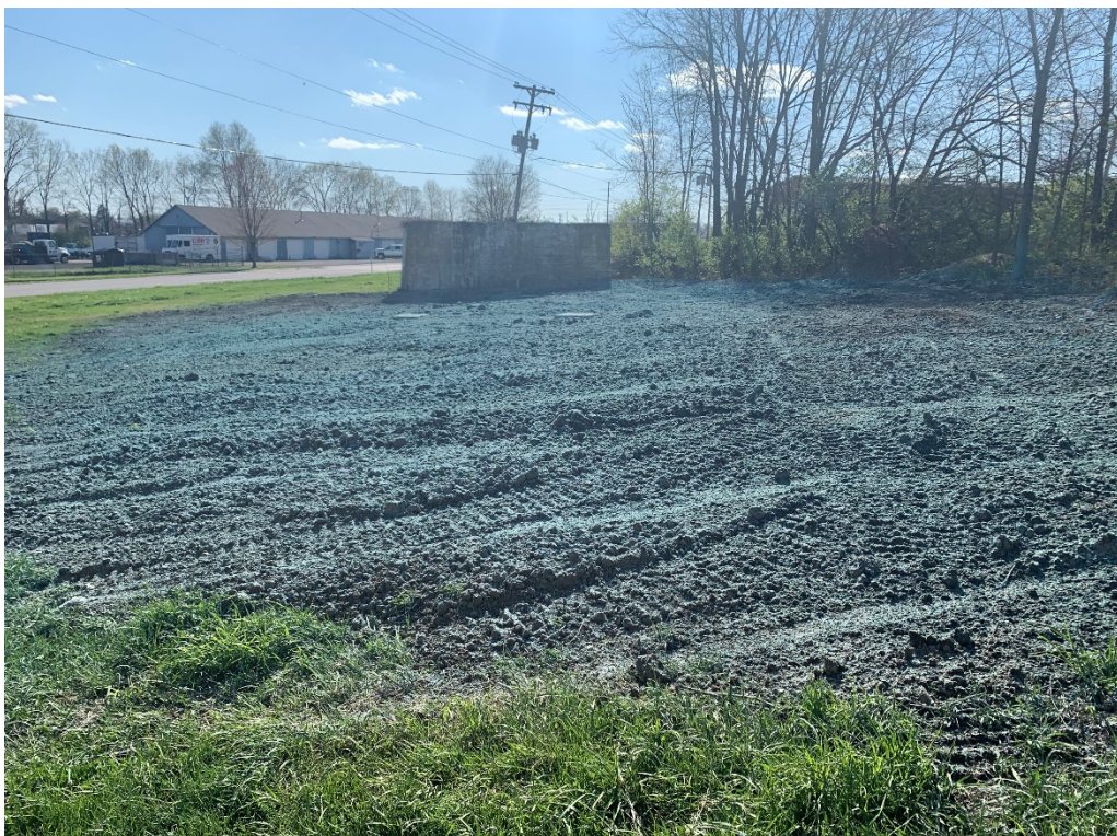
Photo 24: Final grade with hydroseed looking west (April 10)
