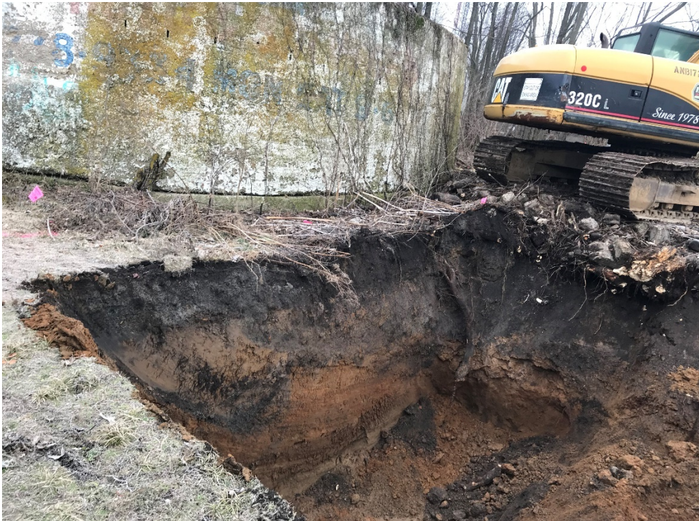
Photo 3: Begin excavation adjacent to concrete cylinder (February 12)
