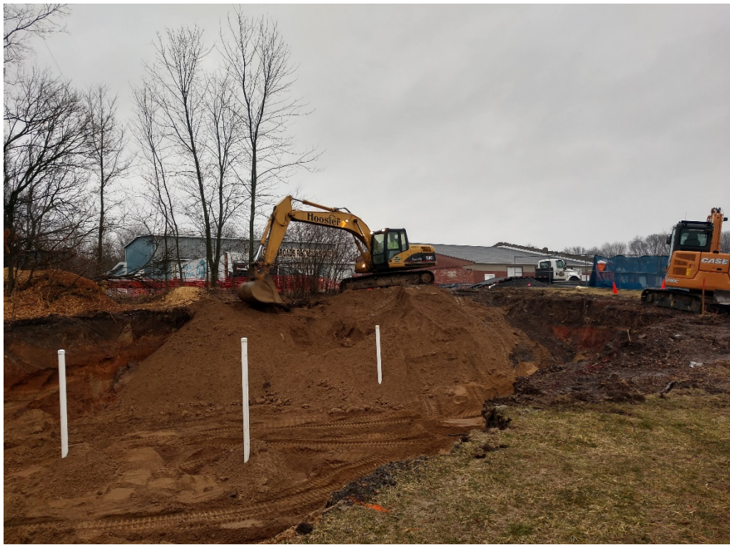
Photo 16: Beginning of backfill (February 24)
