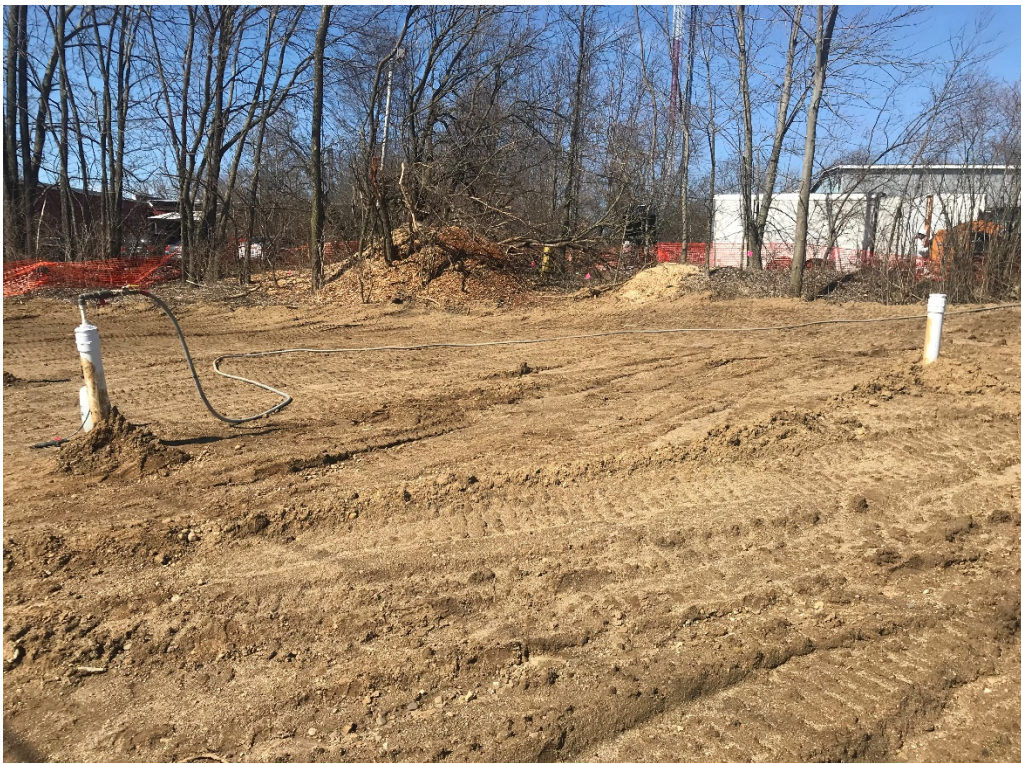
Photo 22: Injection hose hooked up to injection line (March 4)
