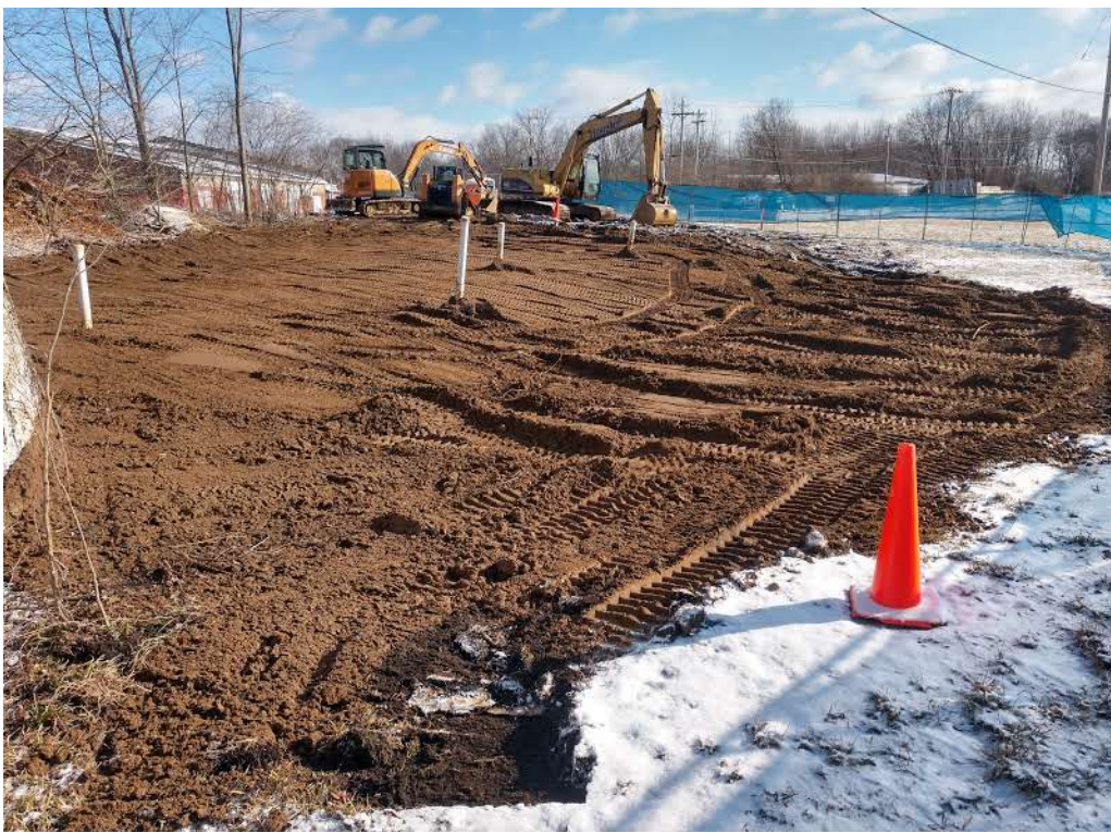
Photo 20: Completed backfill of excavation area (February 27)
