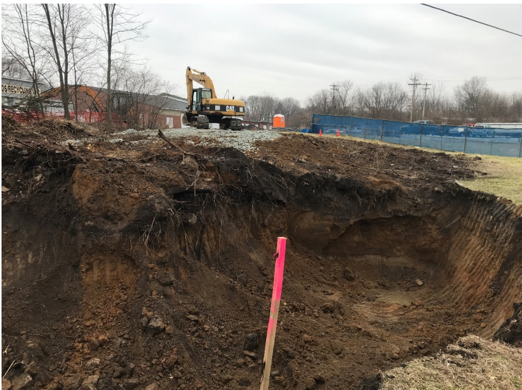
Photo 4: Soil removed as of end of day on February 12
