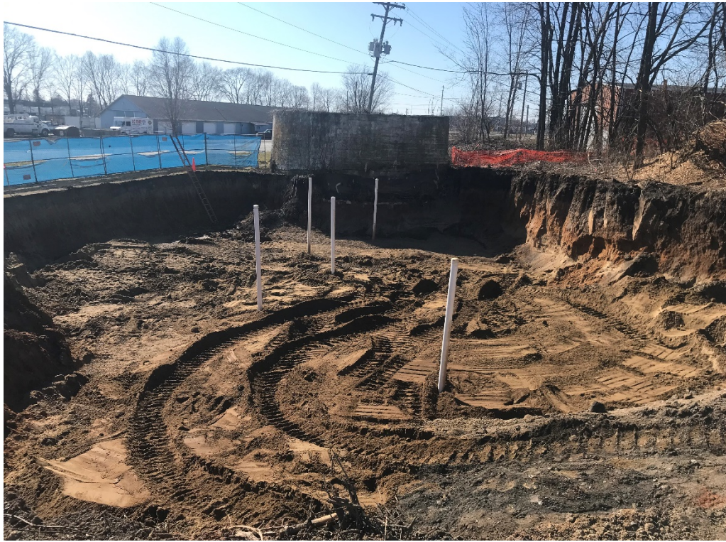
Photo 15: Infiltration Gallery injection lines placement completed (February 21)
