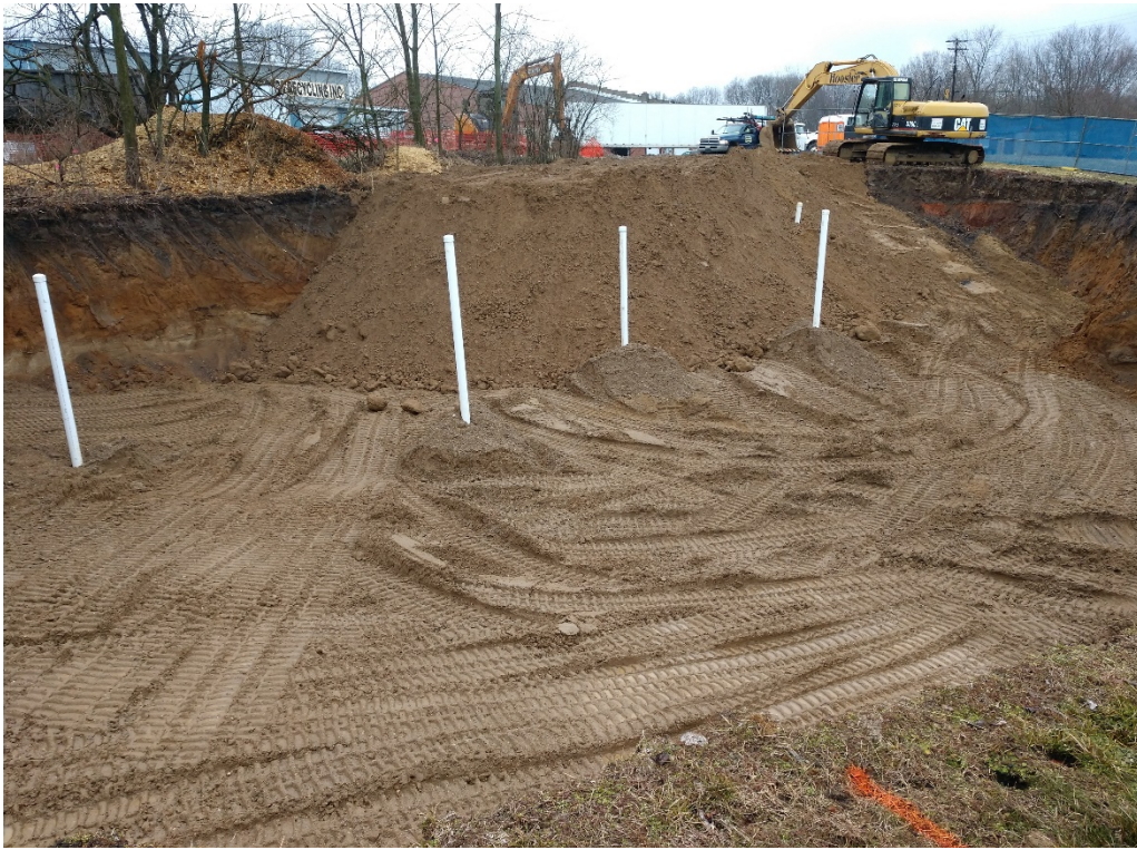
Photo 17: Mounded soil around injection lines for stability during backfill (February 24)
