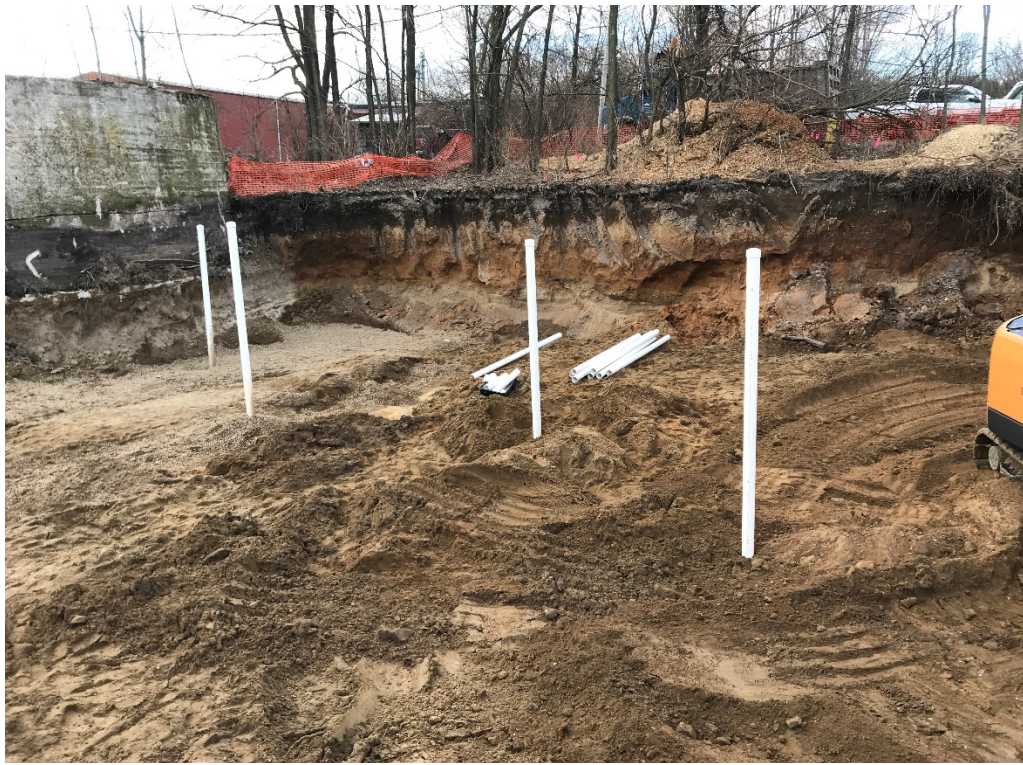
Photo 13: Injection Lines 1-4 completed (February 20)
