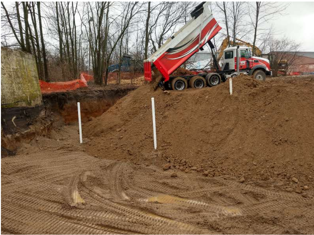
Photo 18: Backfill extending to the western edge of excavation area (February 25)
