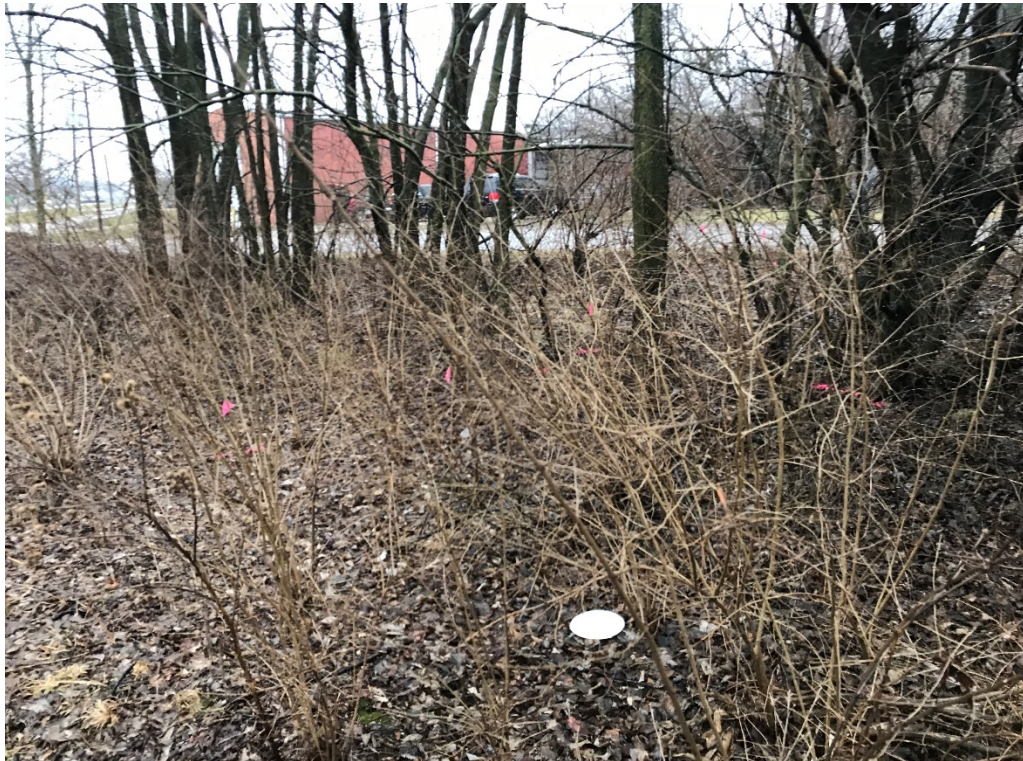
Photo 1: Trees/foliage in excavation area prior to removal (February 10)
