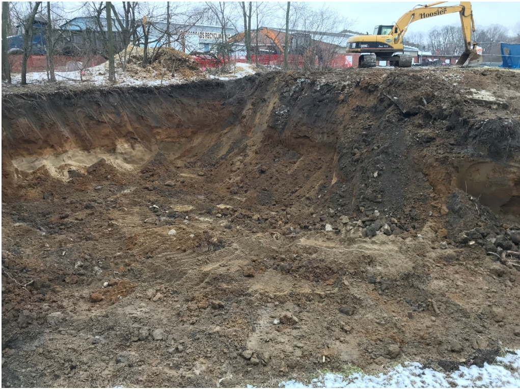
Photo 5: Continued excavation (February 13)
