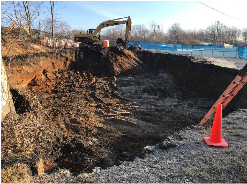
Photo 9: Completed excavation area (February 19)
