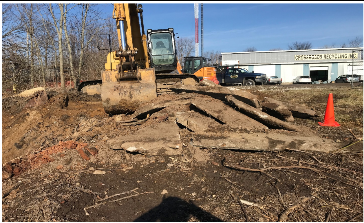
Photo 10: Broken concrete slabs removed from eastern side of excavation area (February 19)
