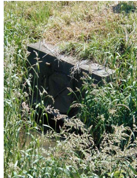
COMBINED SEWER OVERFLOW
