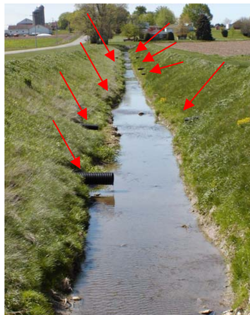
Field tiling along newly constructed ditch
