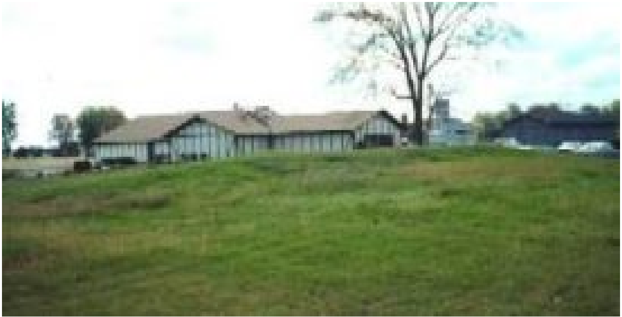
FIGURE 9: MOUND SYSTEM Notice the elevated sand mound on-site system in this person's yard. Mound systems are one way to overcome some limitations. Photo courtesy of Purdue University
