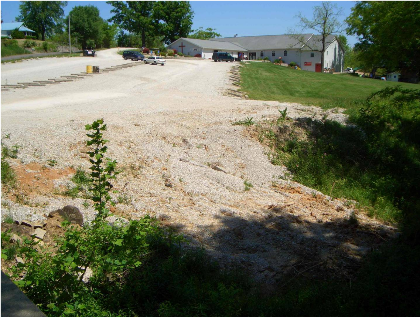
FIGURE 49: SEDIMENT ENTERING JACK’S DEFEAT CREEK. In the foreground, gravel and soil from this church parking lot are washing down the bank to Jack’s Defeat Creek.
