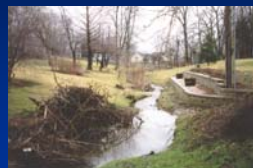
Floodplain encroachments constrict flow and increases downstream erosion
