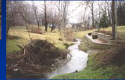
Floodplain encroachments constrict flow and increases downstream erosion
