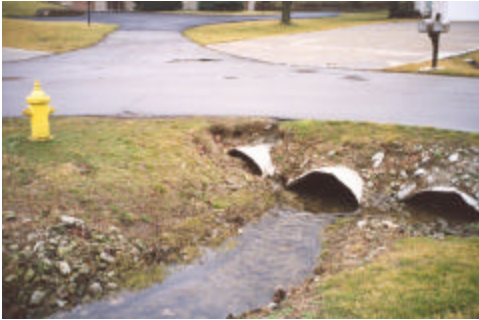
Culvert in Need of Sediment Cleanout
