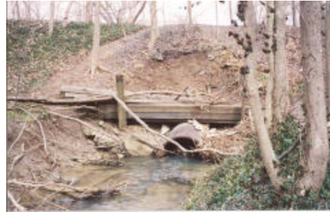
Culvert Pipe Collapse and Erosion
