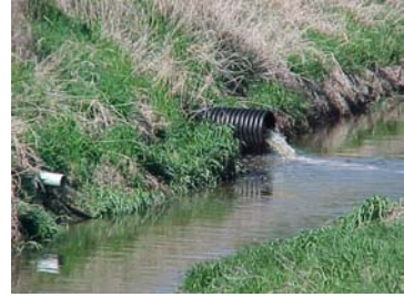
Figure 19 Field tiles discharge into a ditch in the watershed. Photo courtesy of St. Joseph River Watershed Initiative.
