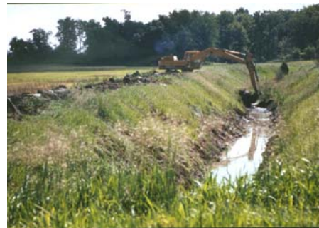
Figure 34 Dipping of ditches removes built-up sediment and vegetation from the bottom of the stream. The spoils placed along the side of the ditch and often creates a negative flow barrier between the stream and the ditch. Photo by Karen Griggs, 2003.
