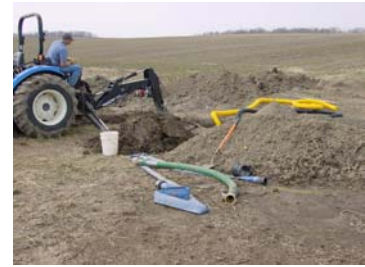
Figure 17 Field depression tile system installation in the SWPI project area, spring 2005. Photo by Jane Loomis.
