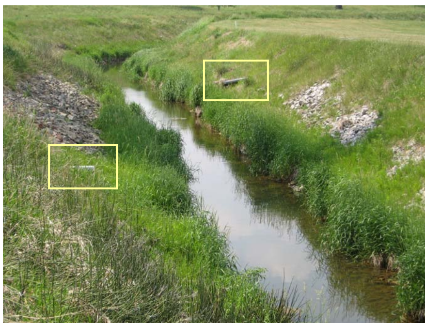
Figure 29. Tile Drains in the Duck Creek Watershed
