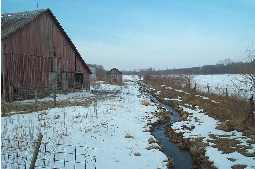
Shackelford Ditch at County Road 450 East (downstream). Note bank trampling and sloughing due to livestock grazing.
