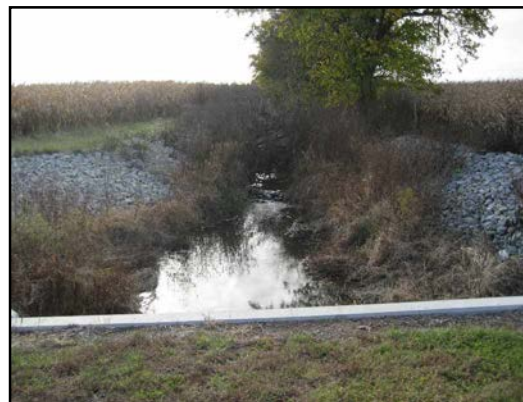
Example of Rip-Rap Stabilized Streambank
