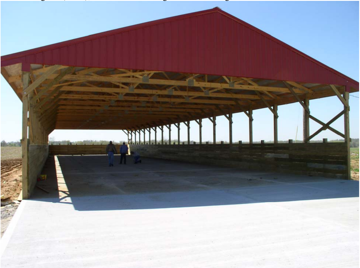
Photo 1. Manure Staging Facility: Constructed to protect manure from environmental elements which cause the transport of E. coli and nutrients into surrounding lands and water sources. Source: Daviess County SWCD July, 2005.
