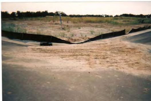
Figure 54. Representative erosion and runoff from construction sites in Salt Creek watershed (2006)
