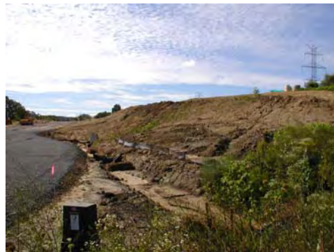
Figure 55. Representative erosion and runoff from construction sites in Salt Creek watershed (2006)
