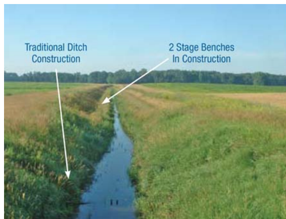
Figure 3-5. Two stage ditch in Northwest Ohio (ODNR 2008b).
