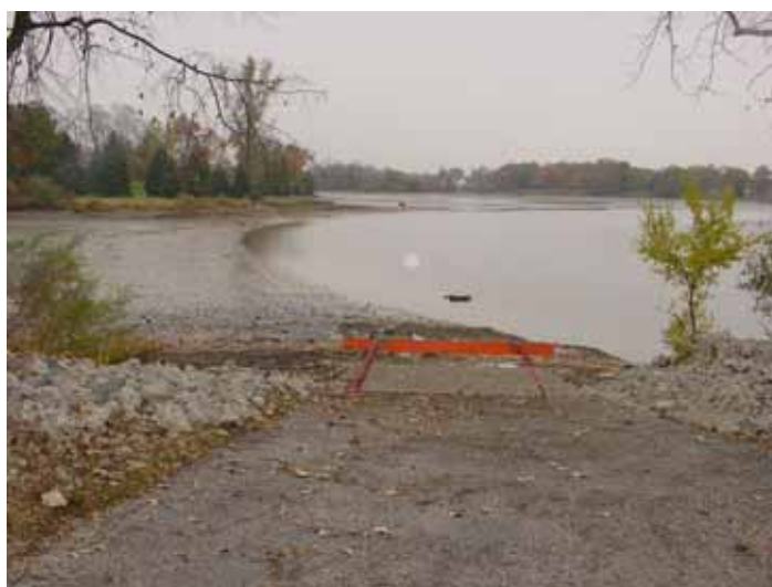
Figure 37 The Cedarville Reservoir was drained in 2006 to facilitate repairs on the dam. (J. Loomis 2006)
