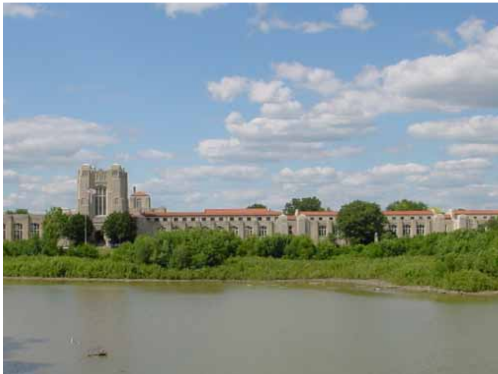
Figure 4 Filtration Plant at the confluence of the St. Joseph, St. Marys and Maumee Rivers in Fort Wayne. (City of FW)
