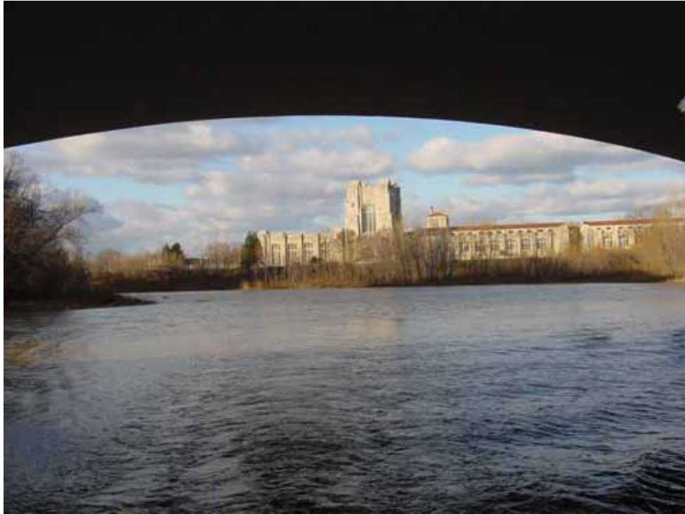
Figure 2 Fort Wayne's Three Rivers Filtration Plant. (J. Loomis, 2005)
