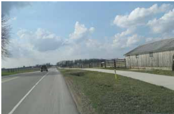
Figure 20 The 0.7 mile Allen-Grabill Community Wetlands Trail includes an extra lane on the highway for Amish buggies. (J. Loomis 2007)
