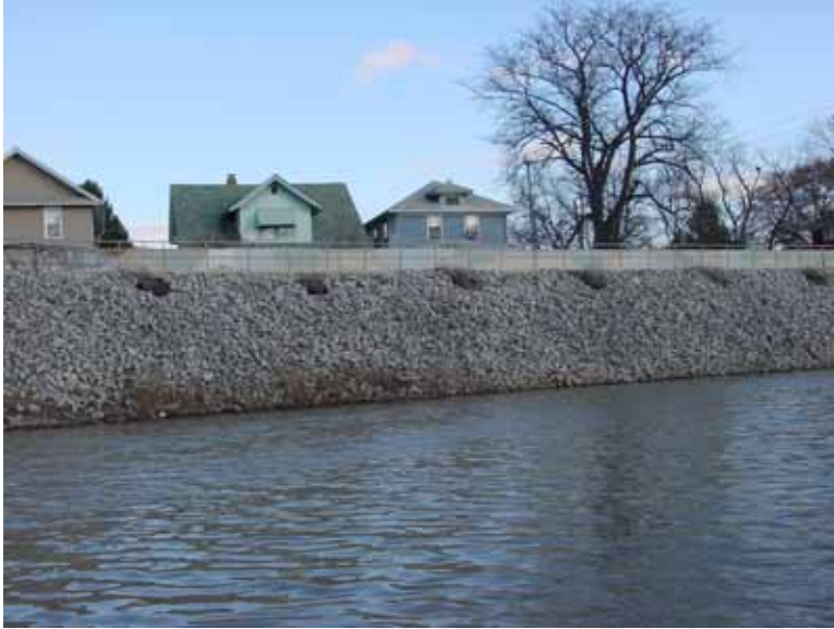
Figure 47 An Army Corps of Engineers flood control project removed vegetation and added rip-rap to the banks of the St. Joseph in the Northside neighborhood of Fort Wayne (J. Loomis, 2005)
