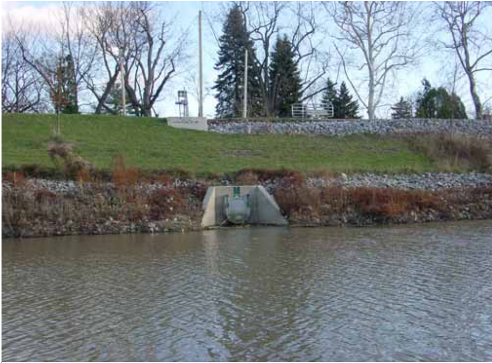
Figure 46 A Combined Sewer Outfall (CSO) on the St. Joseph River in the Northside neighborhood area. (J. Loomis, 2005)
