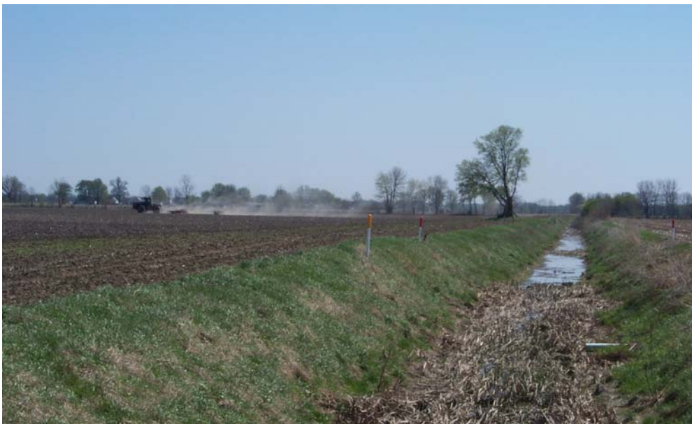
Figure 3.2 Photo of Swanfelt Ditch in northern reaches of watershed exhibiting sedimentation, low flow, water vegetation, no vegetative setback from top of bank, conventional tillage (occurring in photo at time of photograph), and subsurface drainage tiles.
