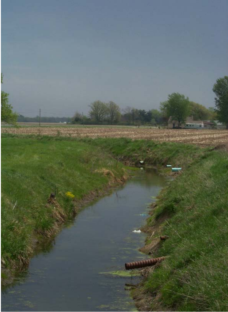
Figure 3.3 Photo of Swanfelt Ditch just south of State Road 28. This photo exhibits no vegetative setback distances from cropping activity, numerous subsurface tile drainage outlets, slow moving water, high algae growth, and a rural residence that uses a septic system on high clay, poorly drained soils.
