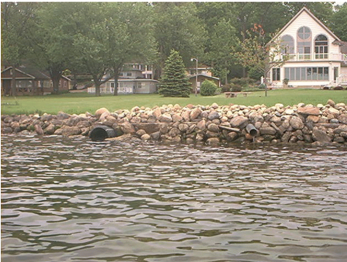
Figure 57. Sample Storm Water Inlet on Lake Tippecanoe
