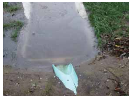
Runoff from parking lot entering stormwater treatment basin at Washington Park
