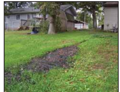
Failing Septic Systems in LaPorte County
