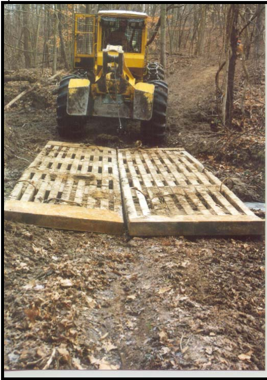
Figure 4.7 (courtesy of Pike Lumber Company, Inc.) – Use of this temporary bridge BMP protects streams and stream banks during logging operations
