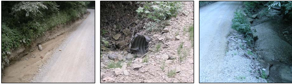
Figure 5.6. Yellowwood Lake Road: Ditch erosion, crushed culverts, and degrading road conditions
